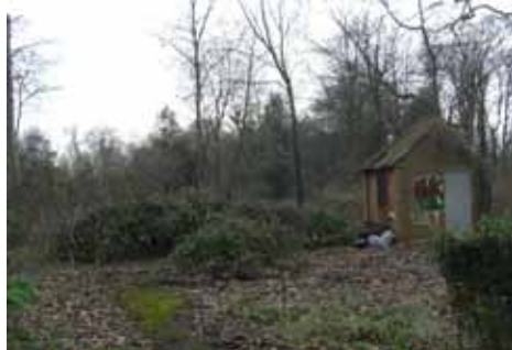
Neglected chalet in Ravensbury Park
