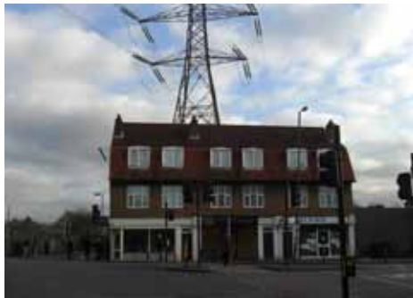
Pylon behind London Road
