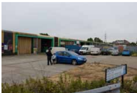
Forecourt in need of enhancement on Church Road
