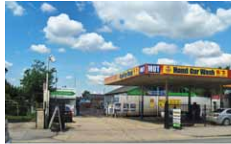
Commercial development along London Road
