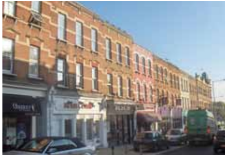
Leopold Road looking east
