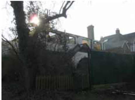
No. 10 Bathgate Road - semi-demolished
