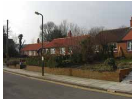
Bungalows in Haven Close
