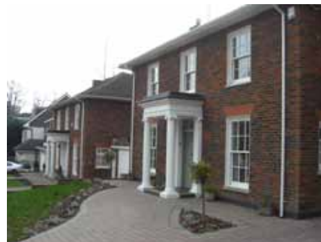
Neo-Georgian houses in Lincoln Avenue
