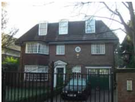
Inappropriate roof alteration with dormers
