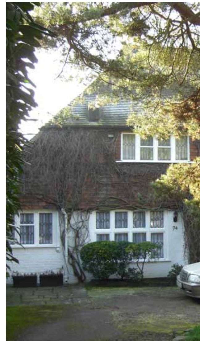
Leaded windows in Bathgate Road
