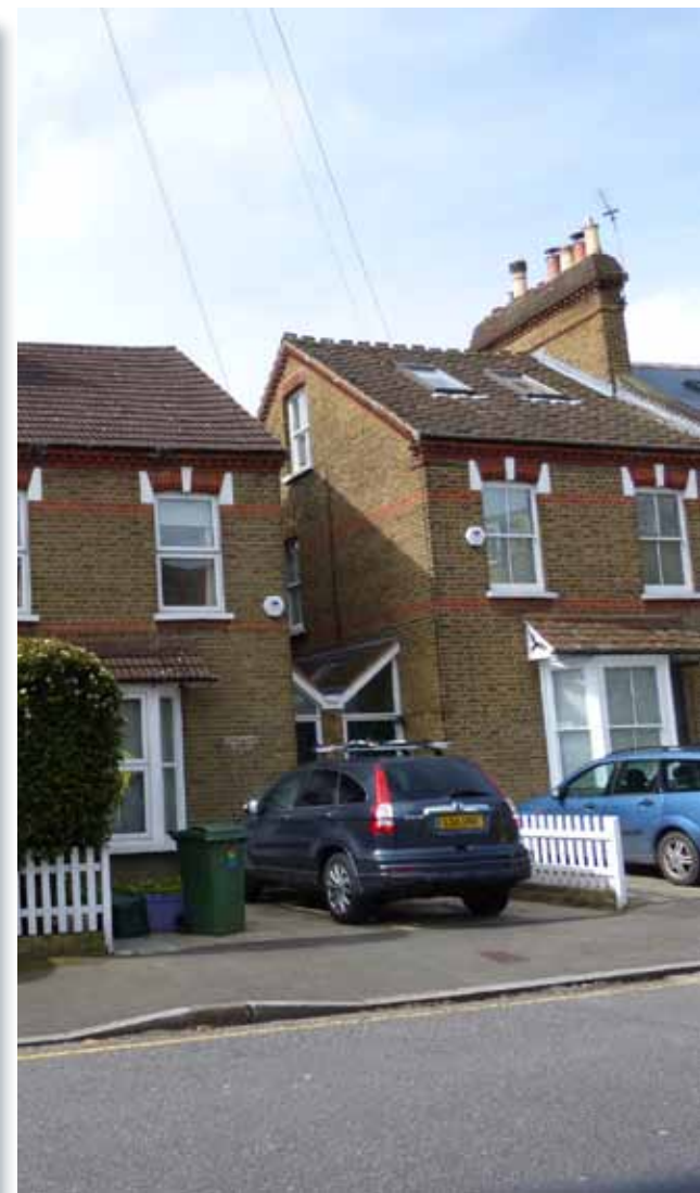
Side entrances on Courthorpe Villas
