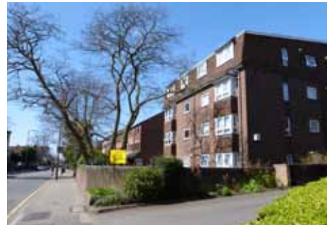
Blocks are set back behind low boundary wall
