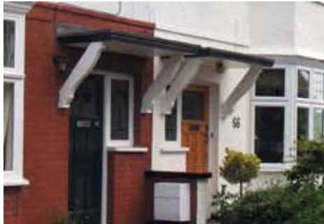
Canopy porch on Camberley Avenue
