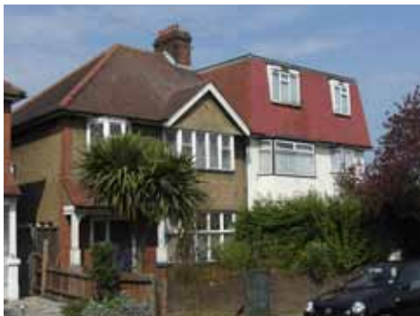
Roof extension Westcroft Gardens
