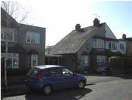
Side extensions in Ashridge Way
