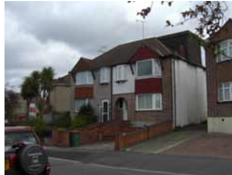
Hardstanding and boundary loss Churlston Drive
