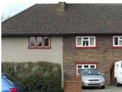
Loss of brick mullions and use of pebbledashing
