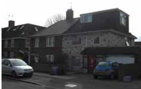
Stone cladding and roof extension
