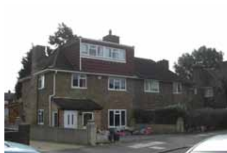
Porch addition and loft extension in Haynt Walk
