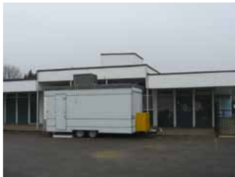
Pavilion at Joseph Hood Recreation Ground
