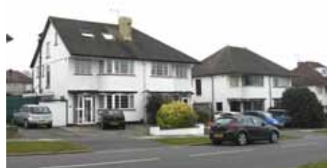
Change of roofline on Cannon Hill Lane
