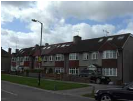
Skylights Churlston Drive
