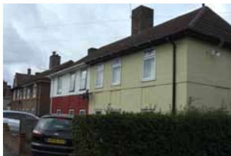
Render and painting of brickwork
