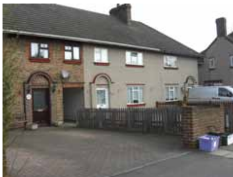
Laying of front gardens to hard standing
