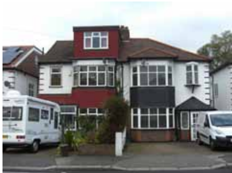
Alterations in Wandle Road
