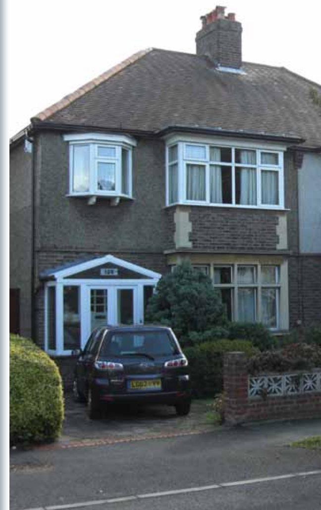
Semi-detached house showing stonework details
