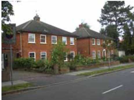
Modern Neo-Georgian semi-detached houses
