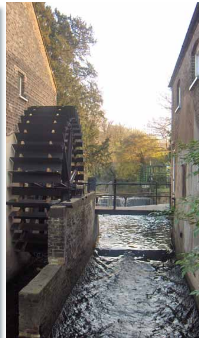
Former snuff mill
