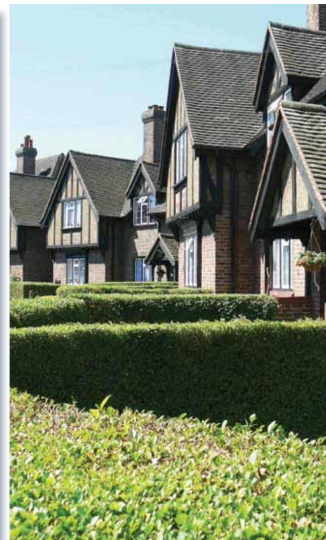
Cottage detailing including gables with timber strapwork and prominent chimneys
