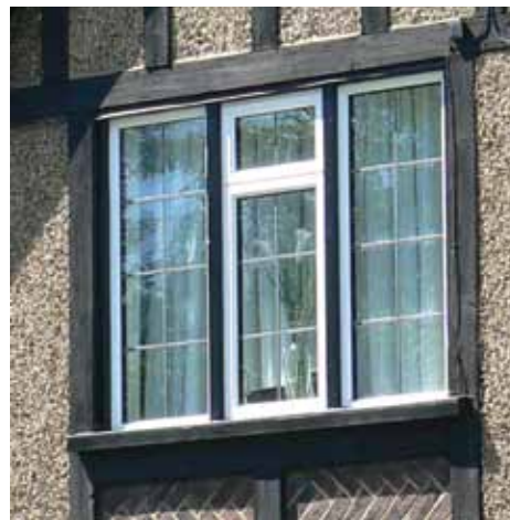
Cottage style windows
