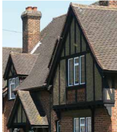
Roofed porches and decorative brick infill panels
