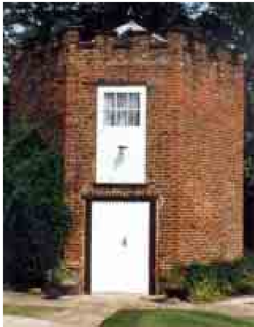
The Listed Observatory Tower Well House
