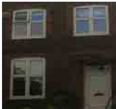
replacement upvc windows at 3 Burghley Road.
