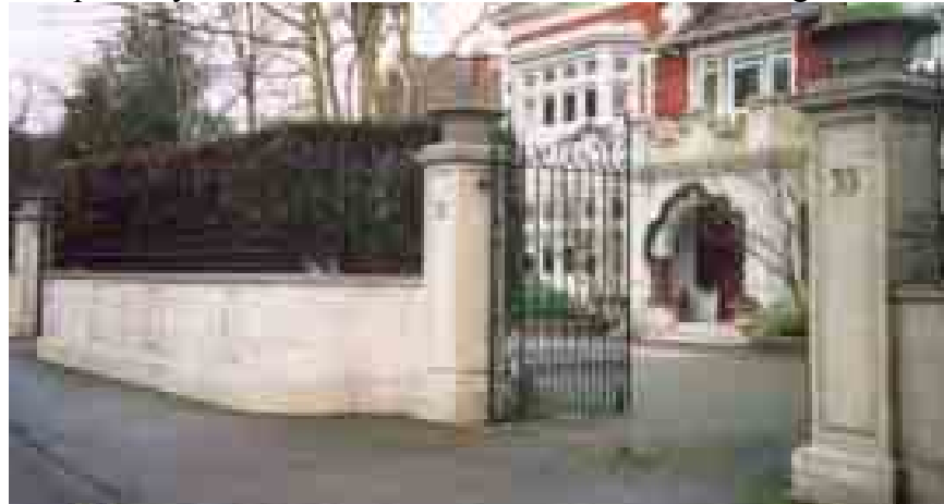
Some boundary treatments in Parkside are of grand appearance
