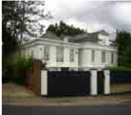
Substantial alterations at No. 29 Burghley Road
