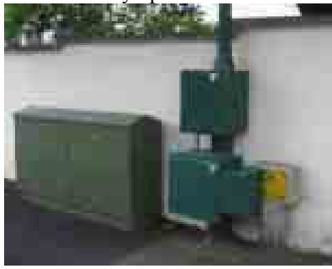
eg. cable installations in Parkside Avenue
