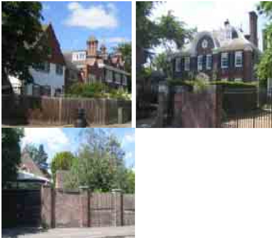
The varied pattern of development on the west side
