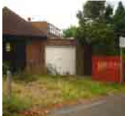
Poor environment at entrance to Dairy Walk and to Wimbledon North Conservation Area
