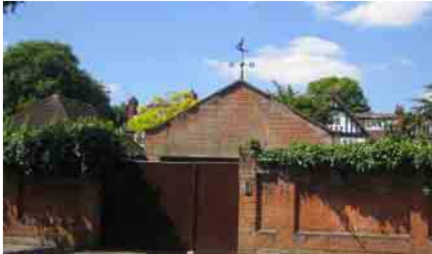
The west side is mostly lined with boundary walls, gateways and ancillary structures to Parkside properties
