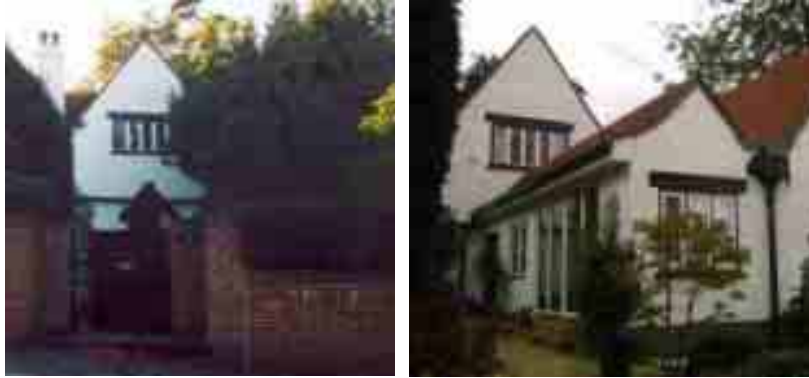
attractive porch and jettied first floor detail obscured by front extension at 27 Burghley Road.
