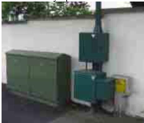
eg. cable installations in Parkside Avenue
