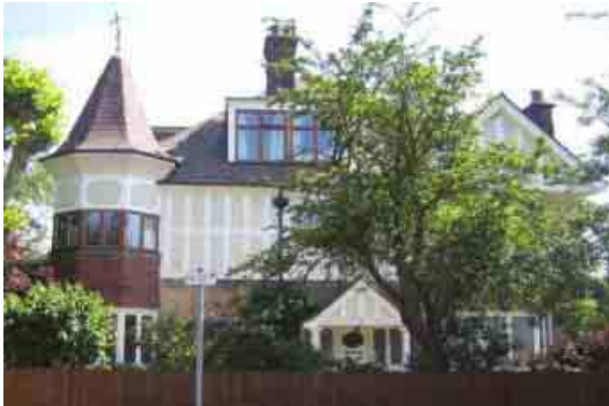
No. 2 Calonne Road
