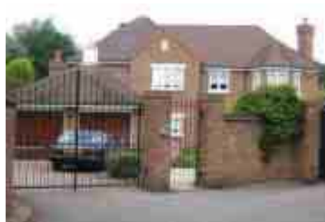
No. 19 Calonne Road
