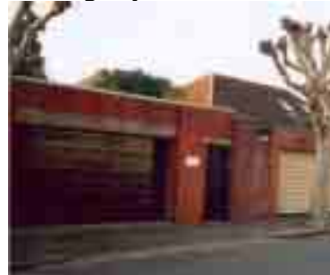
Poor alterations in Parkside Gardens
