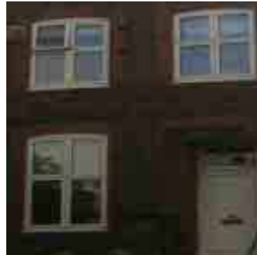
replacement upvc windows at 3 Burghley Road.
