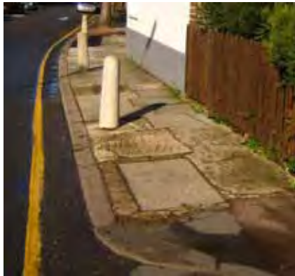
Poor condition of surface and concrete bollards
