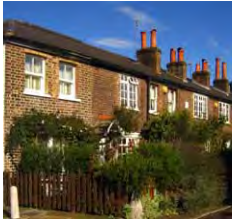
Removal of chimneys
