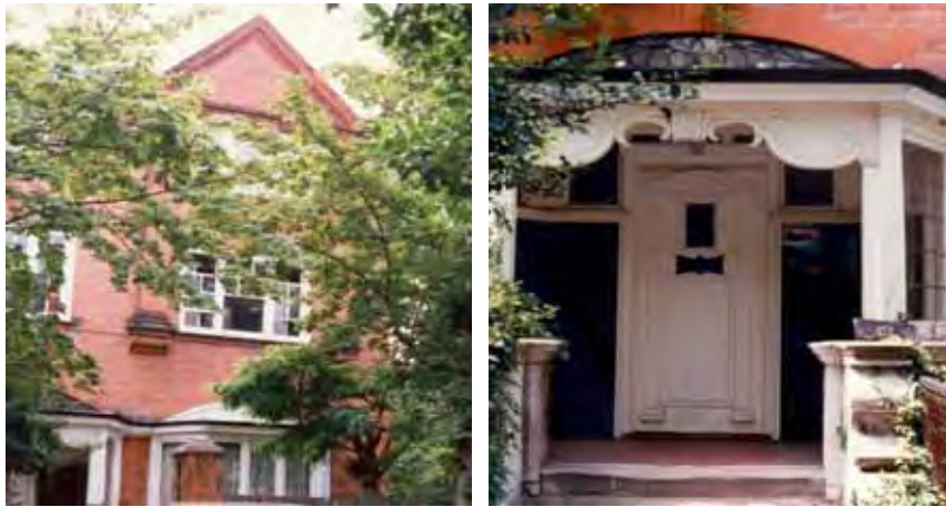
Part of front façade and porch detail at the Listed No. 27
