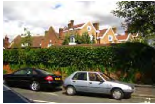
Buildings set back behind high wall on north east side
