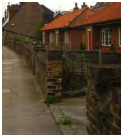
Opening formed within old wall
