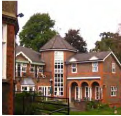
The rear extension at No. 2
