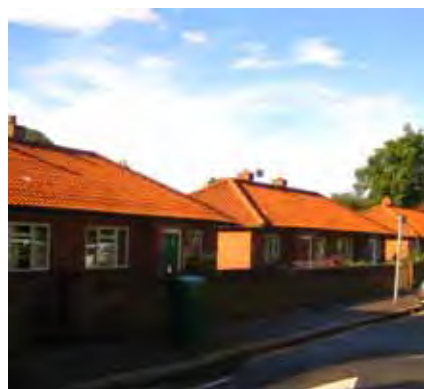
The 1950s bungalows on north west side
