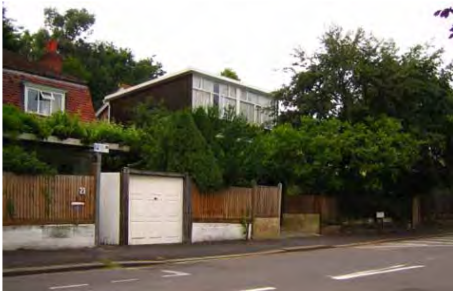
Poor boundaries St Mary's Road Belvedere Drive
