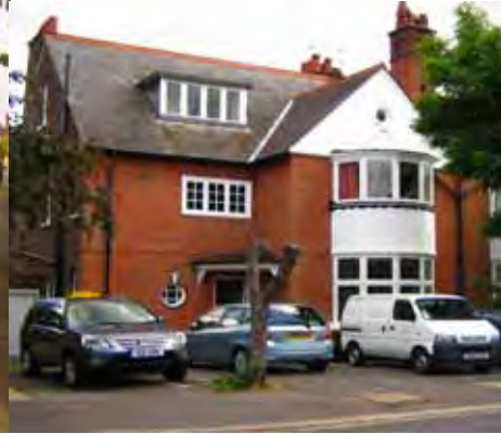
Hardstanding involving loss of greenery
