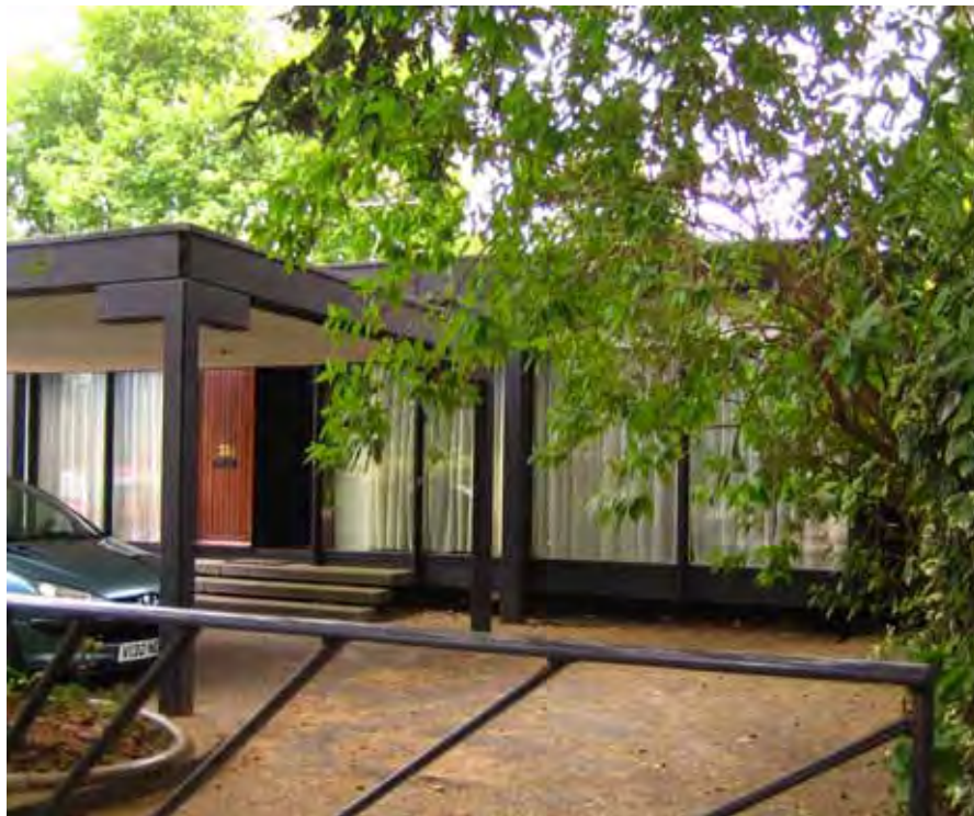
31 b St. Mary's Road, part of a 1960s infill development
