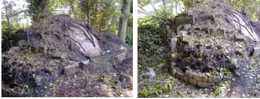
The Ice House exterior
