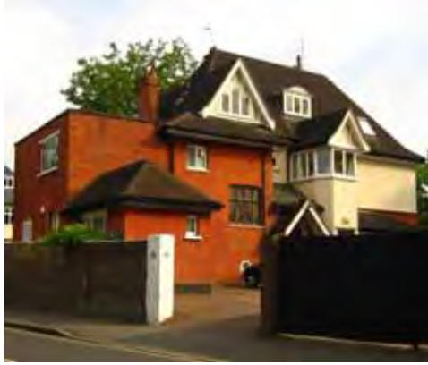
Poor extension, 31 St Mary's Road
