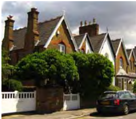
Painting of brickwork can be harmful where brick is the common material
