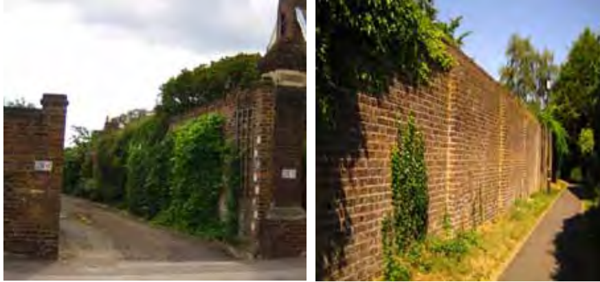
Old brick walls between properties
