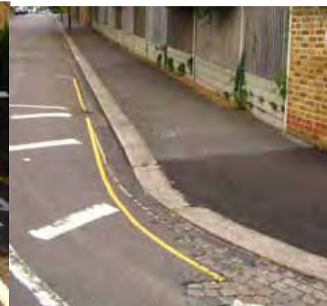
Concrete fence components, covered granite setts
