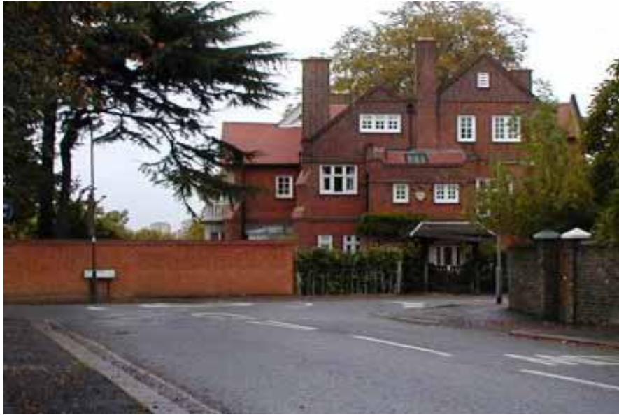
View north to the Listed Building at 61 Arthur Road
