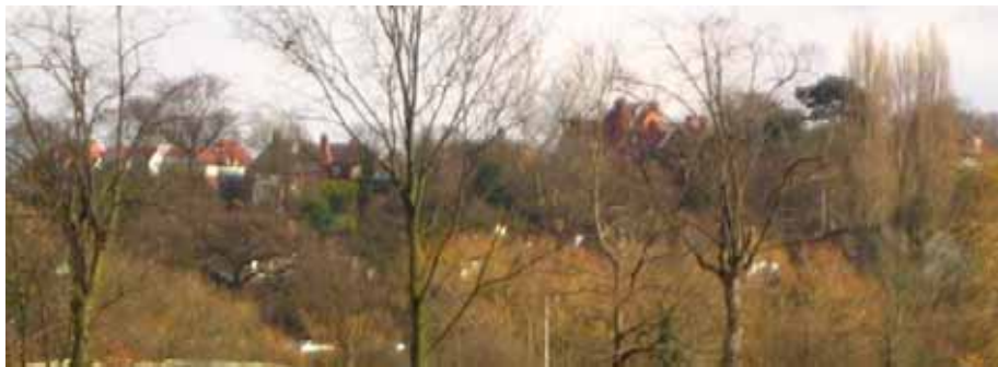
Arthur Road buildings form part of wooded backdrop to Wimbledon Park
