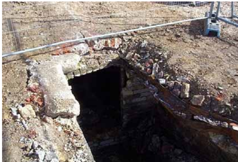
Excavation works reveal tunnel.
