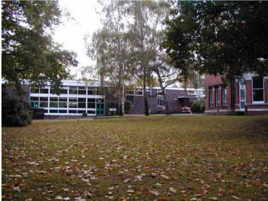
The open setting of the school buildings, from Lake Road
