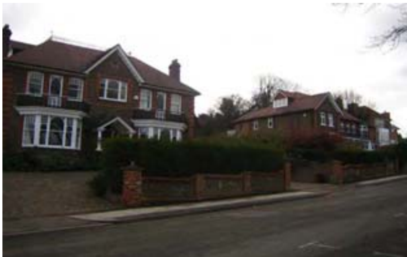
Locally Listed Buildings and their highway boundary
