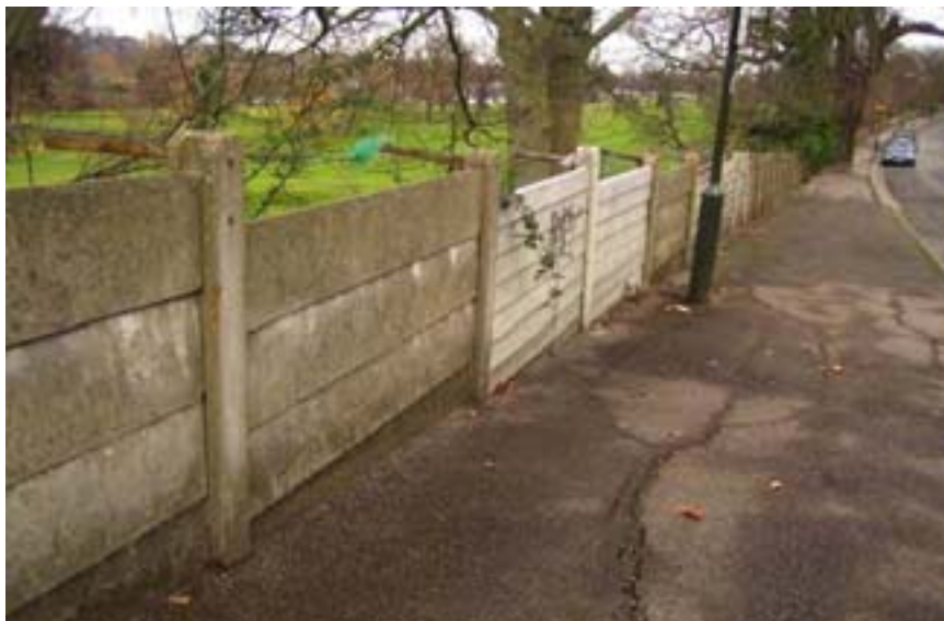
Concrete wall to golf course boundary
