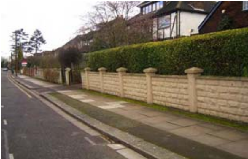
Typical front boundary wall, Home Park Road
