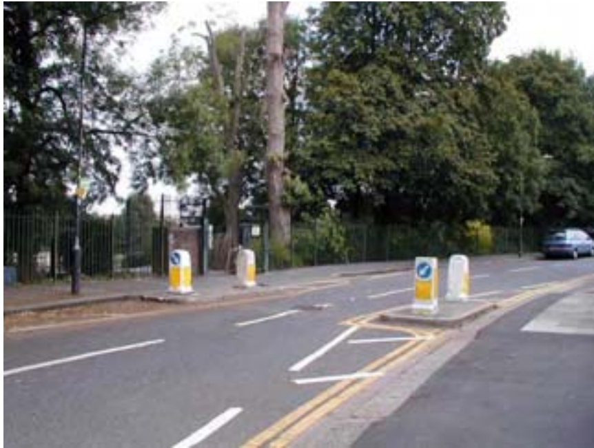
Road narrowing, Home Park Road
