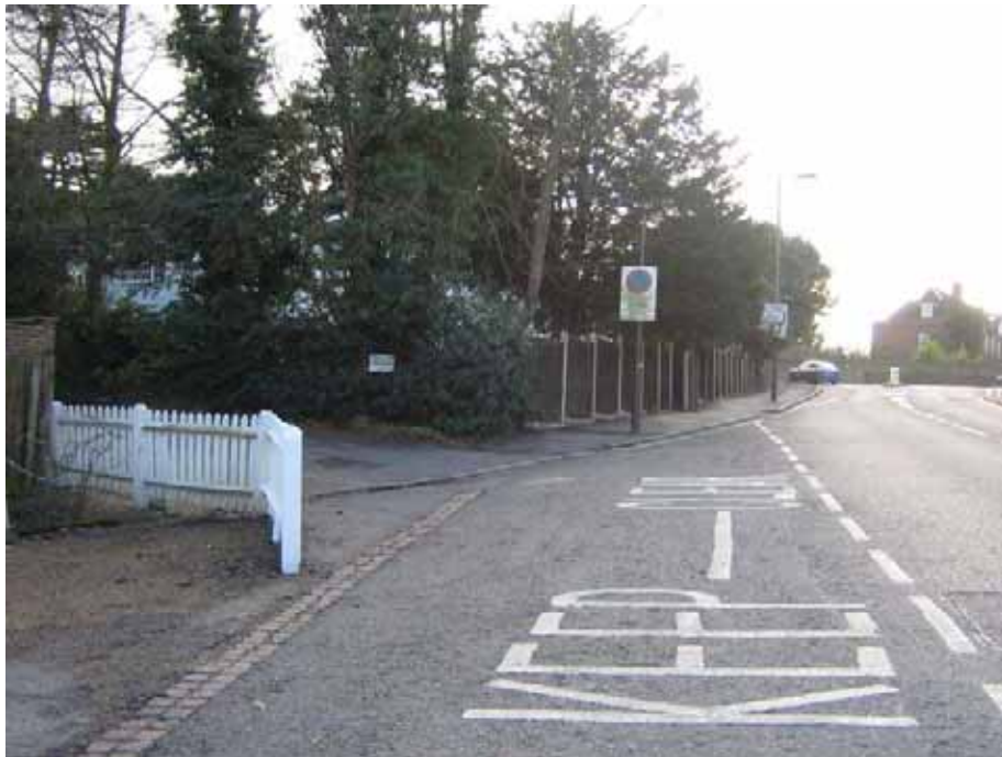
Intrusive road marking in Church Road
