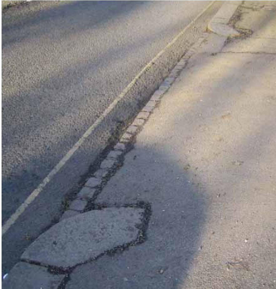
Kerb stone in Arthur Road
