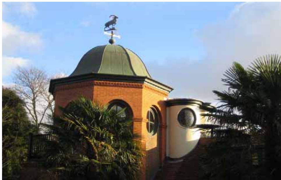
Detail of No.2 Arthur Road
