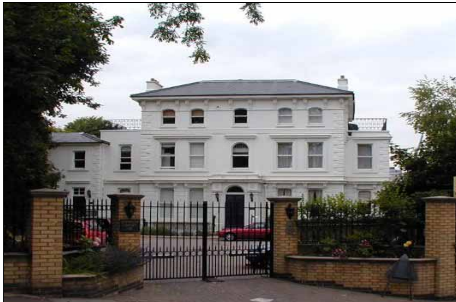
No. 157 Church Road (Renshaw Court)
