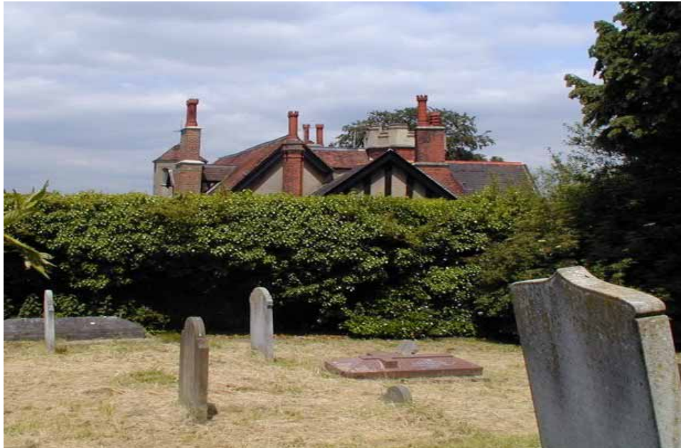
View of The Old Rectory House from within the Churchyard
