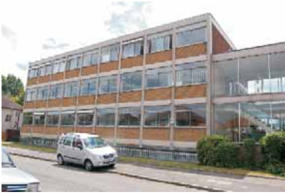
House, 10 Morden Road are also pretty unsightly and detrimental to the character of the conservation area.
