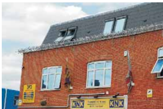
The site is also dominated by the large temporary buildings that have been installed within its curtilage.
