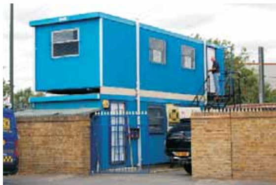
Barons walk, part of which forms the westerly boundary to this part of the conservation area is lined with concrete panel fences to the London Road Playing Fields and metal palings to the adjacent Waste Recycling depot. This
