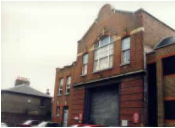
c) Merton Bus Garage - Wandle Bank frontage building.
