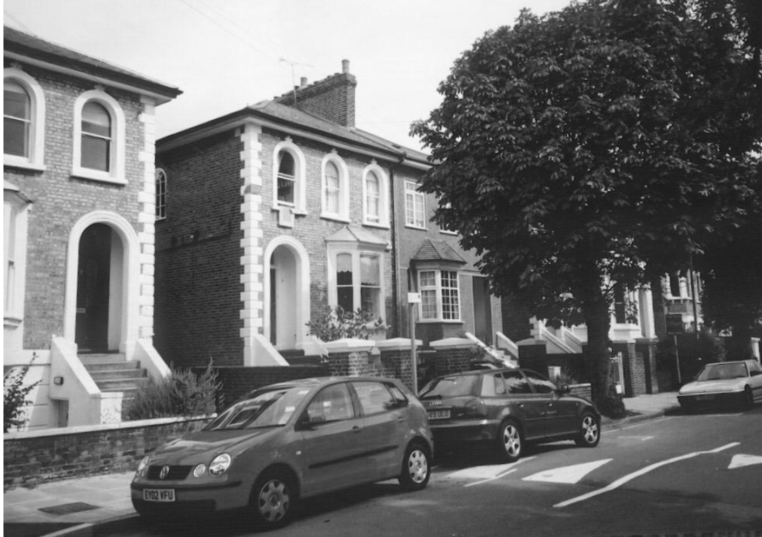
The streetscape to Nos 19 to 23 Pelham Road, indicating its general character (with the exception of the unfortunate alterations to No. 19), of pollarded trees, brick front boundary walls and brick piers, and the shallow gardens dominated by the light-wells to the semi-basements and the steps up to the front doors.
