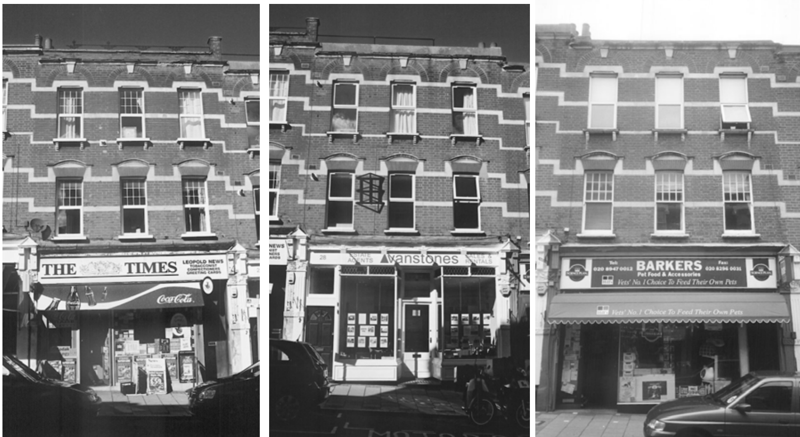
NOS. 30, 28 AND 26 LEOPOLD ROAD. Below: Historic features which have been retained.
