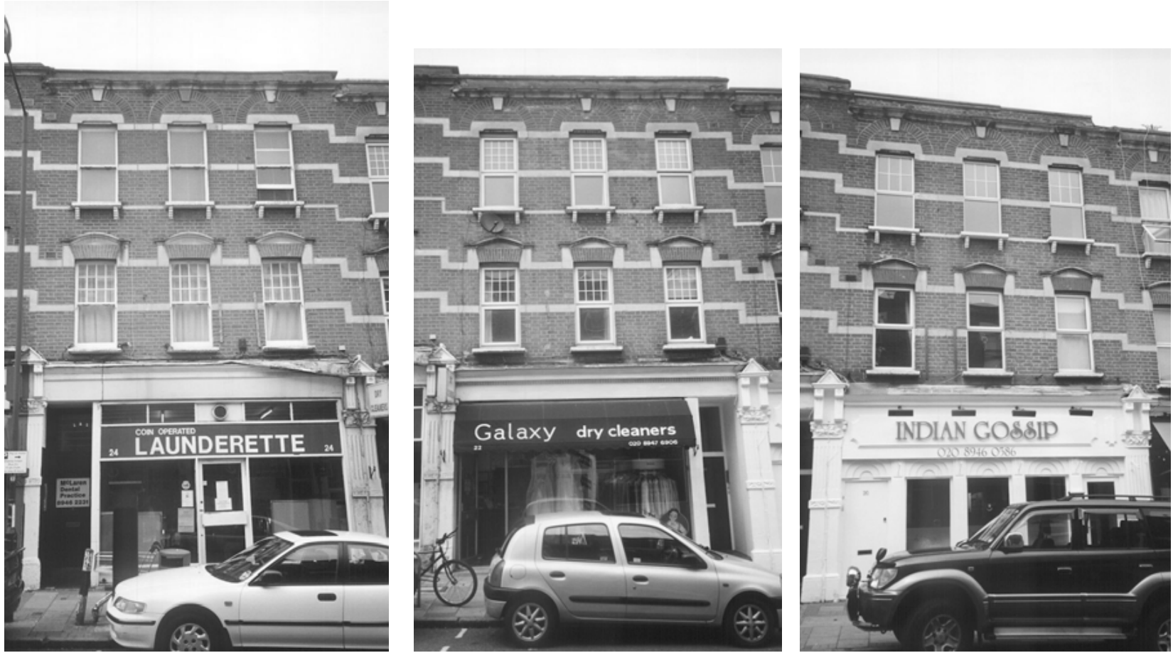
NOS. 24, 22 AND 20 LEOPOLD ROAD. Below: Historic features which have been retained.
