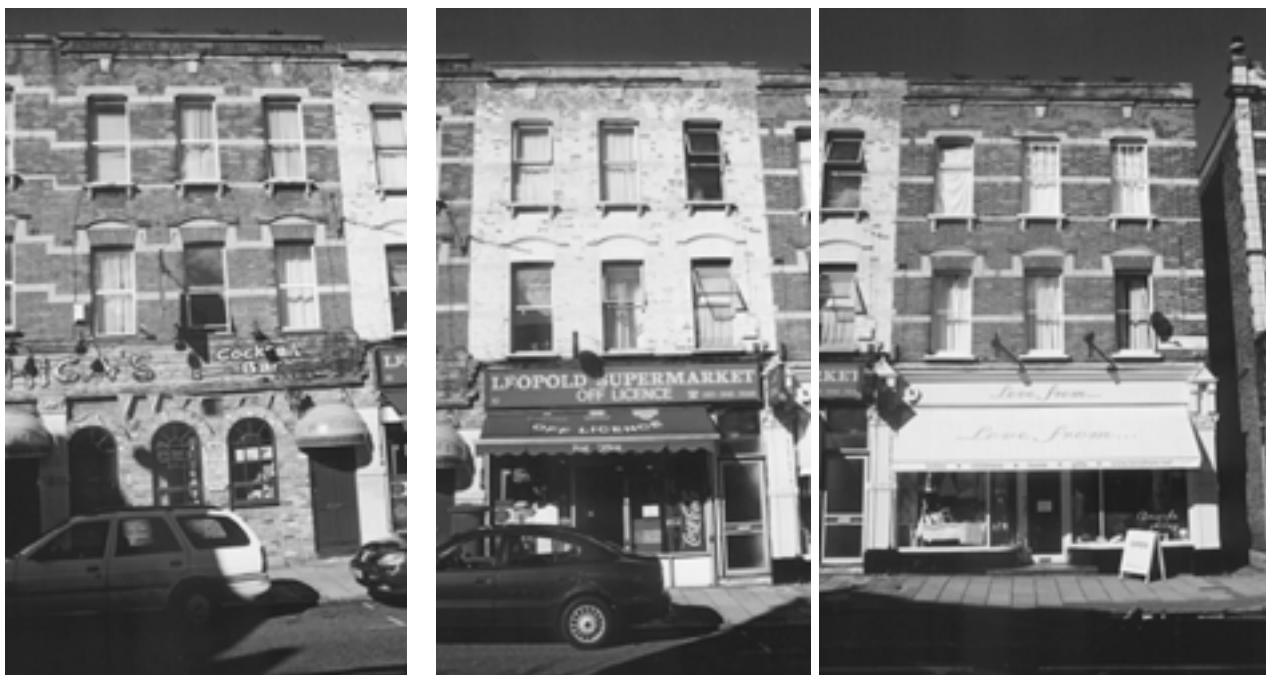
NOS. 12, 10 AND 8. LEOPOLD ROAD. Below: historic features which have been retained.
