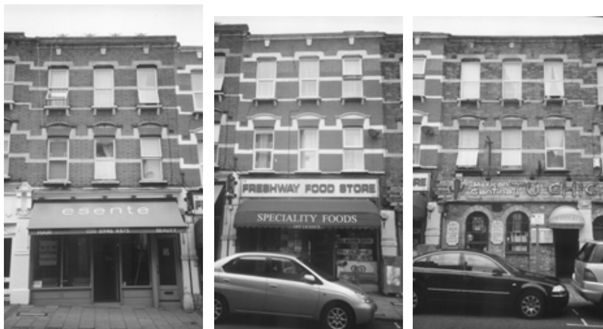
NOS. 18, 16 AND 14 LEOPOLD ROAD. Below: Historic features which have been retained.
