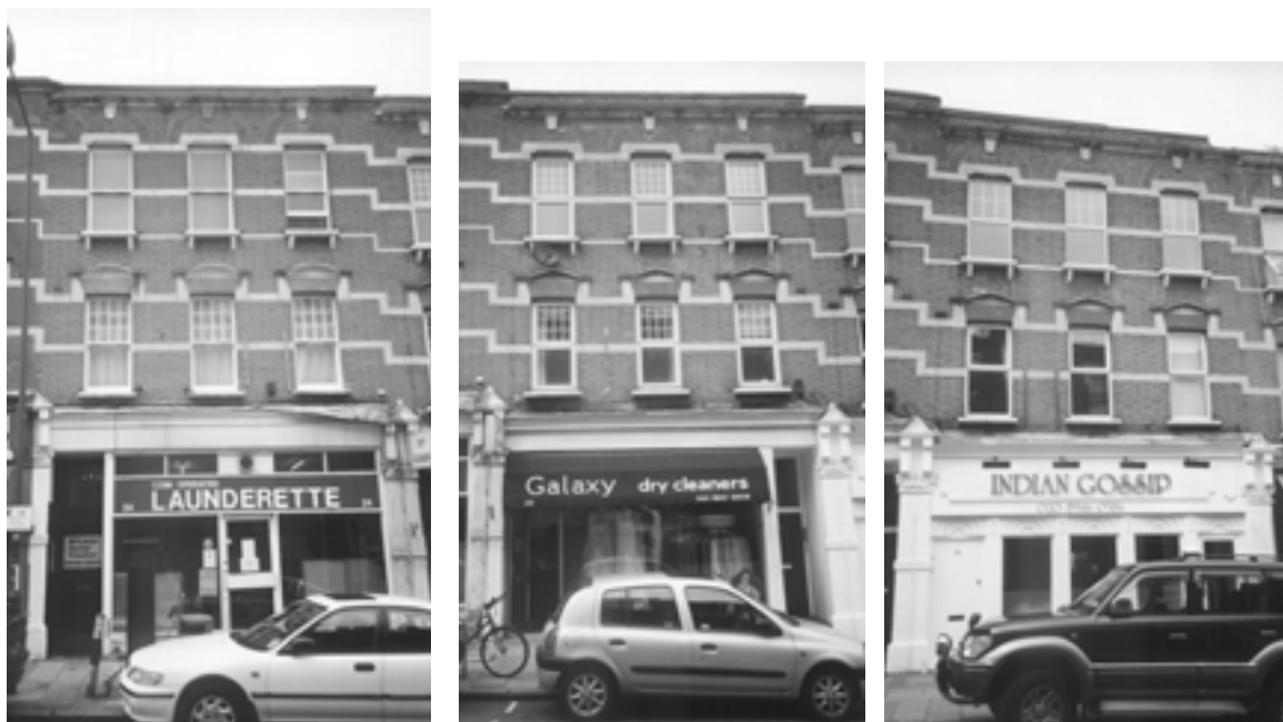
NOS. 24, 22 AND 20 LEOPOLD ROAD. Below: Historic features which have been retained.
