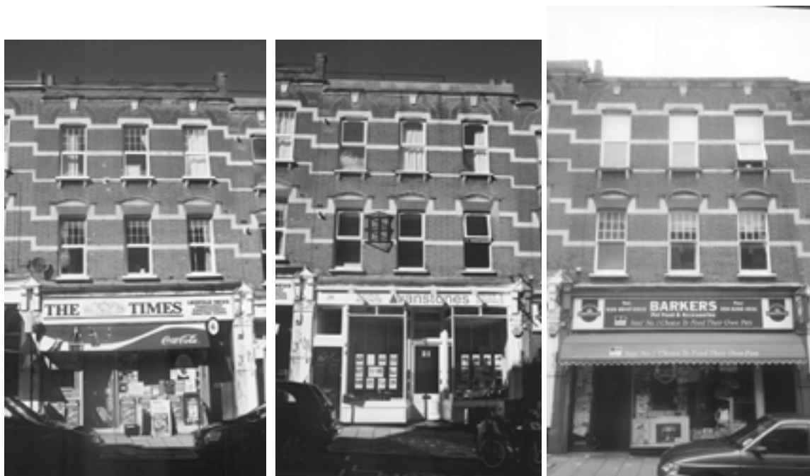
NOS. 30, 28 AND 26 LEOPOLD ROAD. Below: Historic features which have been retained.
