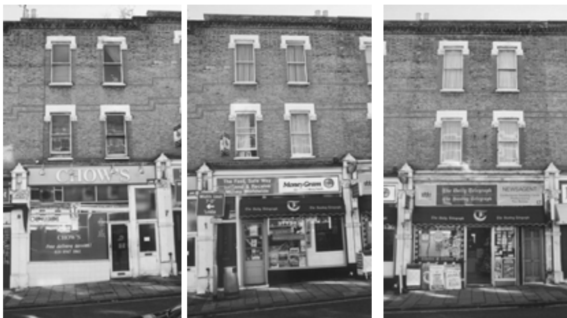
Nos. 13, 15 and 17 Leopold Road. Below: Historic features which have been retained.
