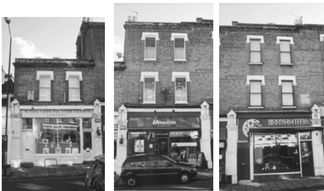
NOS. 7, 9 AND 11 LEOPOLD ROAD. Below: historic features which have been retained:
