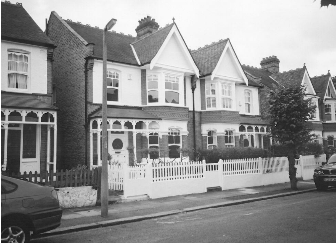
Nos. 29 and 31, showing the typical details of projecting gables, ornamental windows and door details, the band of tile hanging under the first floor windows, vertical brick slips each side of the first floor bays and brick corner piers to the ground floor bays, and white picket fencing above a low rendered brick wall. A typically pollarded tree is shown in line with the party wall, but the one lining up with the rear access way has been removed to allow a lamppost to be erected.
