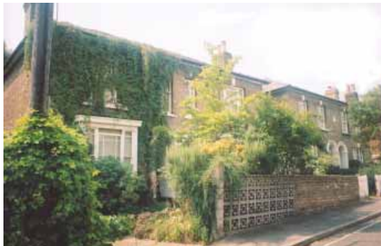
Nos. 33 to 36, showing the unfortunate Trelliswork concrete block wall to No. 33
