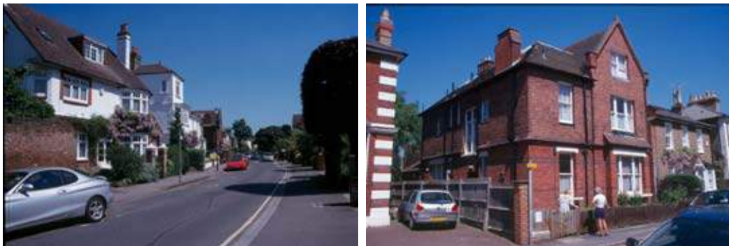
The northern end of Lingfield Road, looking south, and Nos.4 and 5 Lingfield Road
