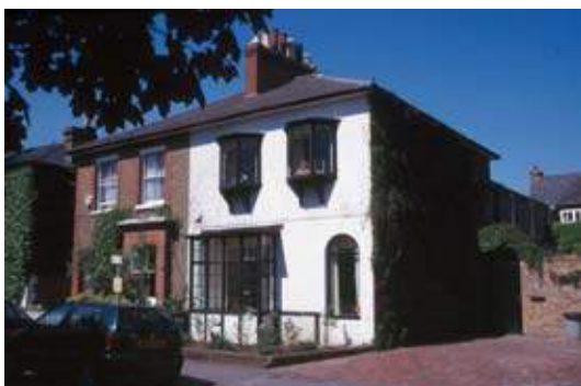
Nos.10 & 11, showing the unfortunate alterations to No.11: white render and unsuitable windows and the recessed car parking space surrounded by a high wall
