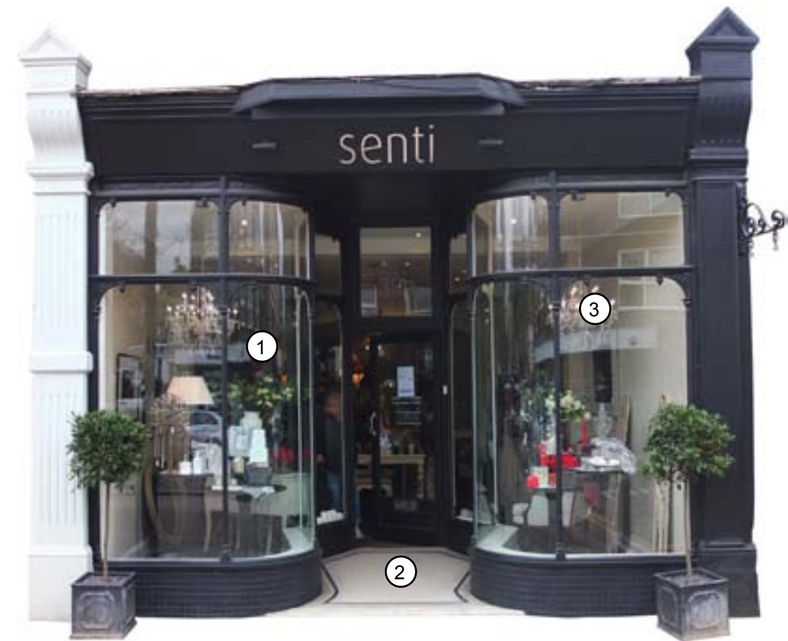
39B Senti Wimbledon ✓ 1. curved glazing makes the display visible from various angles 2. set-back shop door creates dramatic entrance sequence 3. feature lighting in display creates visual interest
