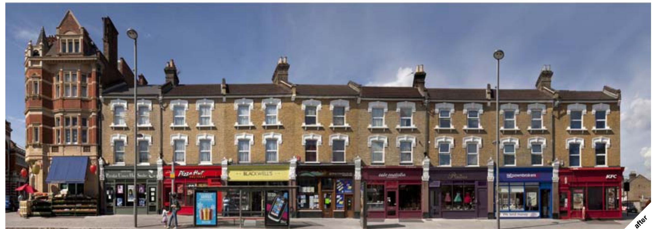
Shop front improvements in High Road Leyton by Jan Kattein Architects
