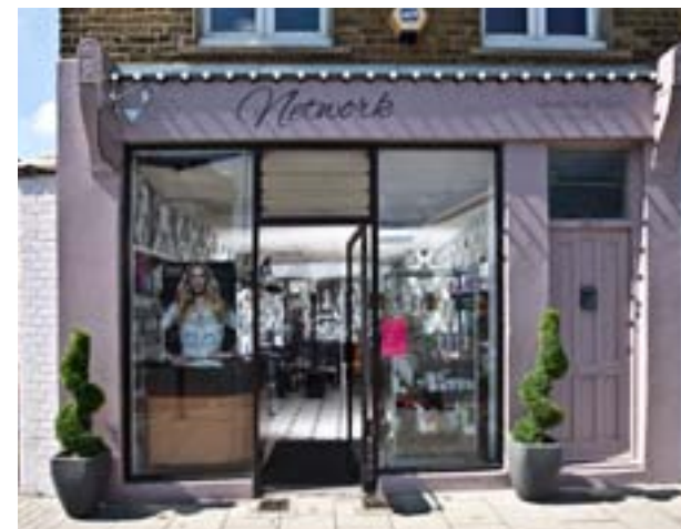
Network in Nunhead has a modern shop front which gives a clear view into the shop. The sign graphics are simple, using two contrasting colours and two fonts. The pots in the forecourt complement the shop front design. A projecting sign is integrated with the fascia sign.
