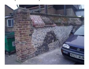
the introduction. repair and/or replacement of flashings or weatherings. minimal descaling, minimal piecing in of stones, replacement of individual stones, facing up damaged stones with mortar 'plastic repairs', application of a surface treatment to consolidate friable areas and treatment of joints including removal of an impermeable cement pointing. Stone repairs should only be undertaken by specialist contractors under the supervision of a conservation professional.
