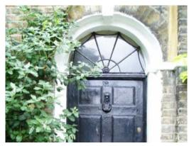
located and local building tradition. The thickness and moulding of glazing bars, the size and arrangement of panes and other details can be indicative of the date of a building and need to be taken into consideration when repairing or replacing windows.
