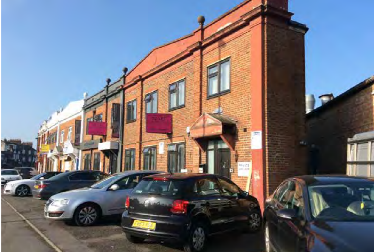
Industrial units fronting Burlington Road
