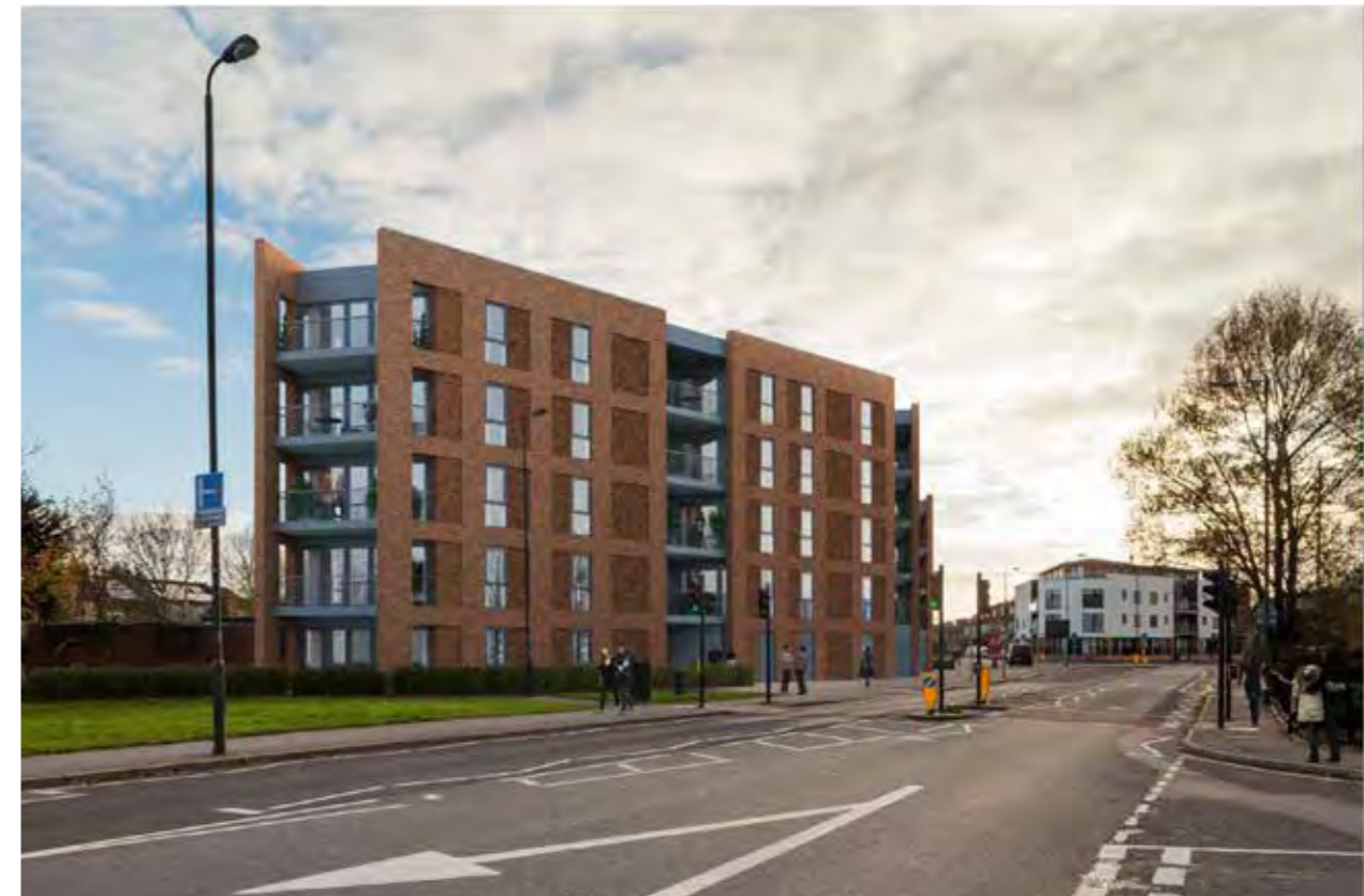
CGI of 5 storey development under construction at Burlington Road
