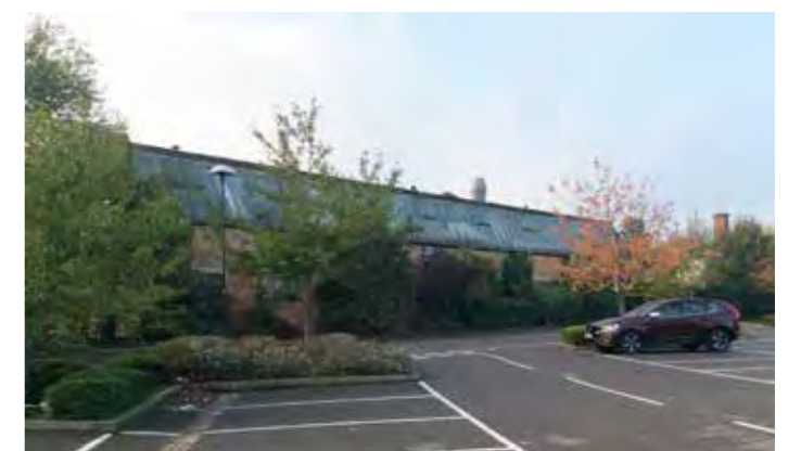
8: Southern site boundary and adjacent industrial buildings
