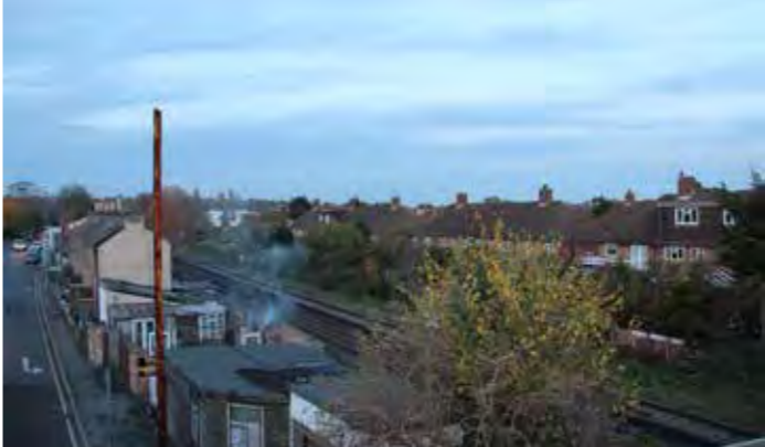
13: View from West Barnes Lane footbridge looking north
