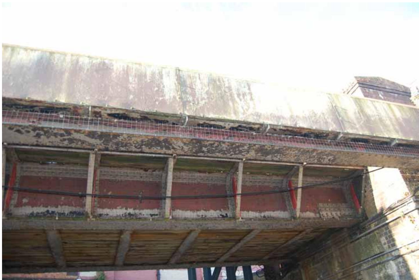
3. View showing algae and soffit requiring repainting
