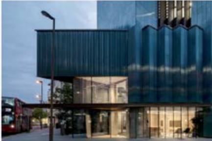
Fig.6.24 - Airlock lobbies in larger buildings provide safety to reduce opportunities for intruders. (Mapleton Crescent, Wandsworth Metropolitan Workshop) [Credit: Simon Kennedy]
