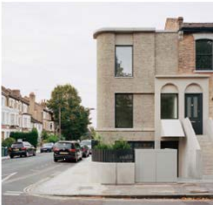
Fig.6.23 - This extension to an existing terrace promotes a sense of security by incorporating defensible space fronting the street. (Corner House, Southwark by 31/44 Architects) [Credit: Rory Gardiner]
