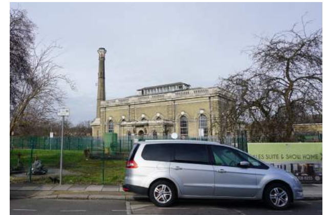
Cricklewood Pumping Station
