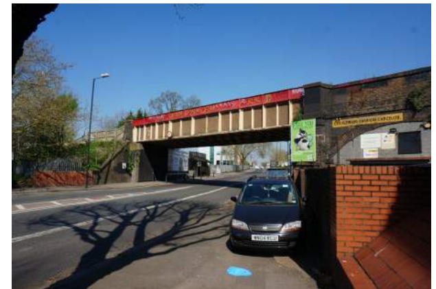
Dudding Hill rail line bridge over Cricklewood Broadway
