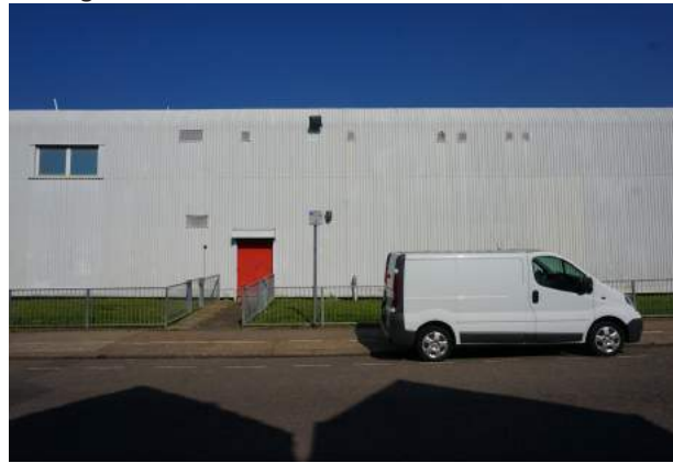
The Matalan store presents no frontage to Temple Road
