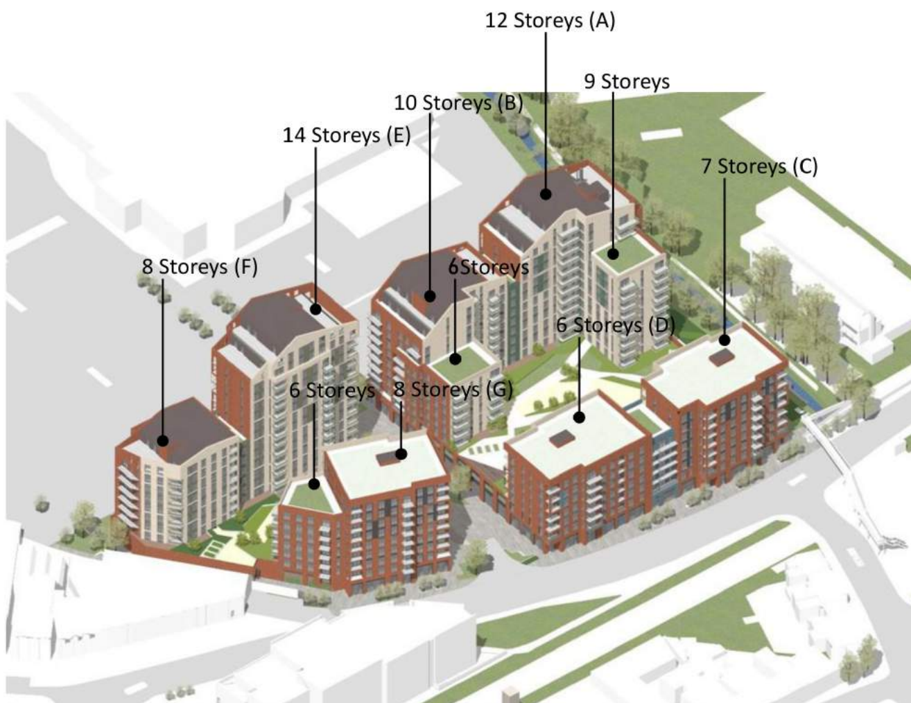
Figure 3.1: Proposed massing of development on Appeal Site taken from DAS Addendum page 5 (storey heights indicated are the number of residential storeys over and above the podium level) (CD/9.3)
