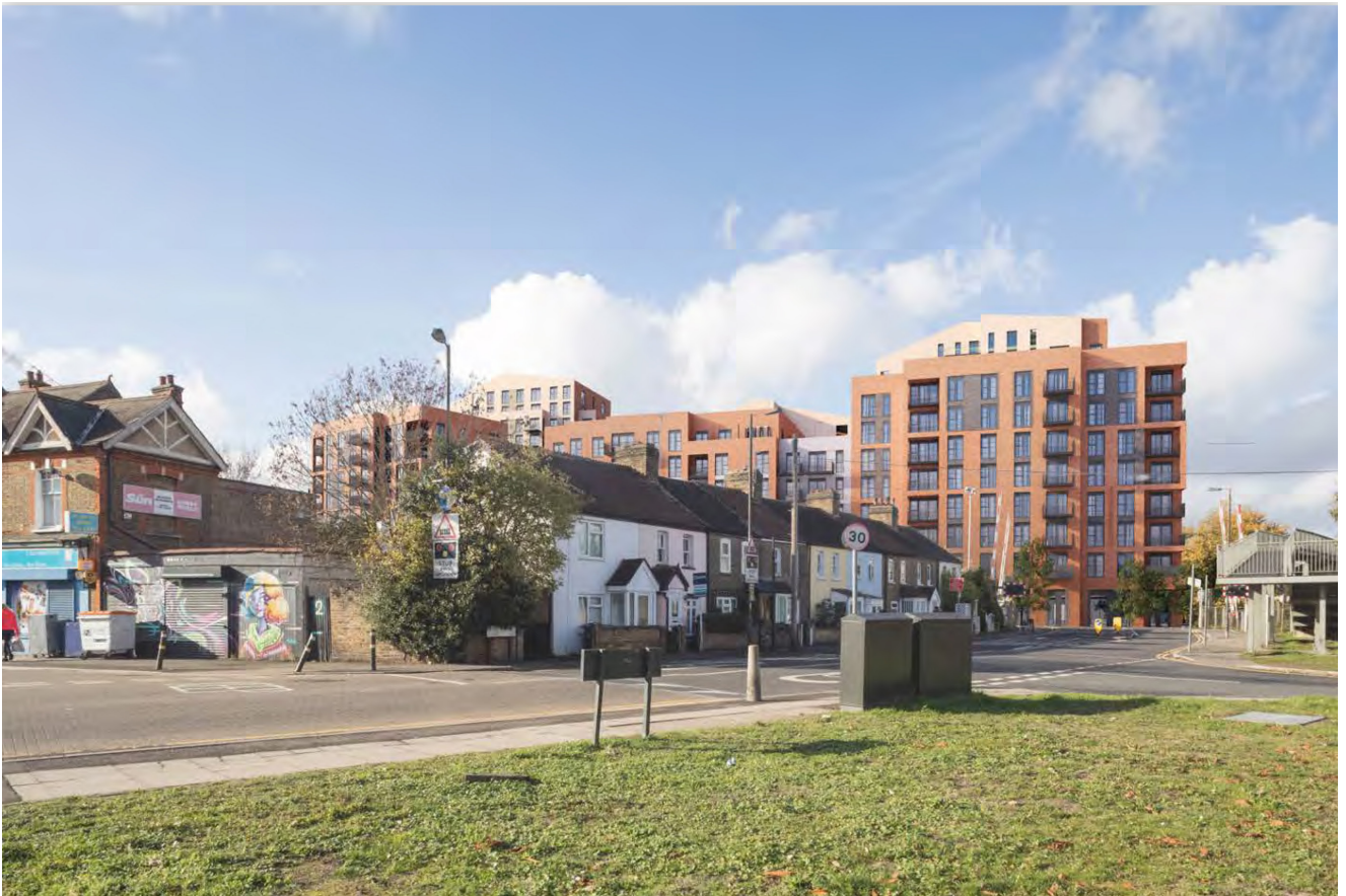
Figure 4.6: View 5 Proposed - West Barnes Lane / Linkway junction from TVA
