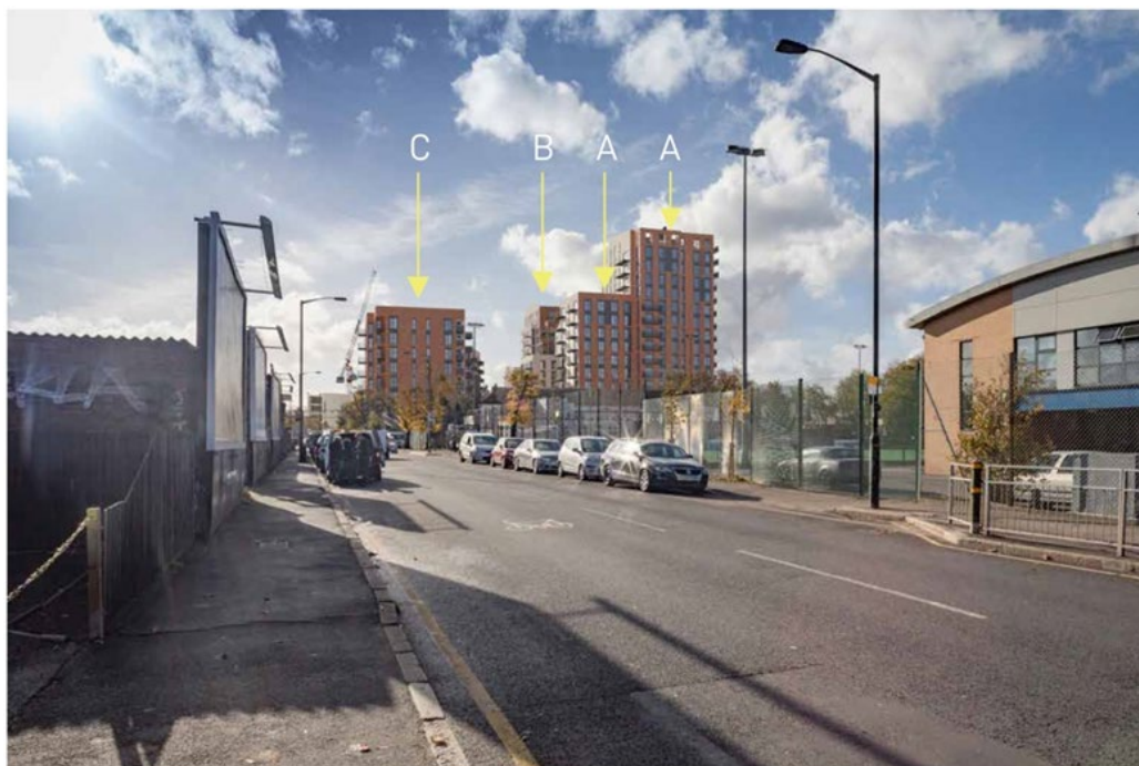
Figure 15: View south along West Barnes Lane – leading to Burlington Road. TVIA View 7.
