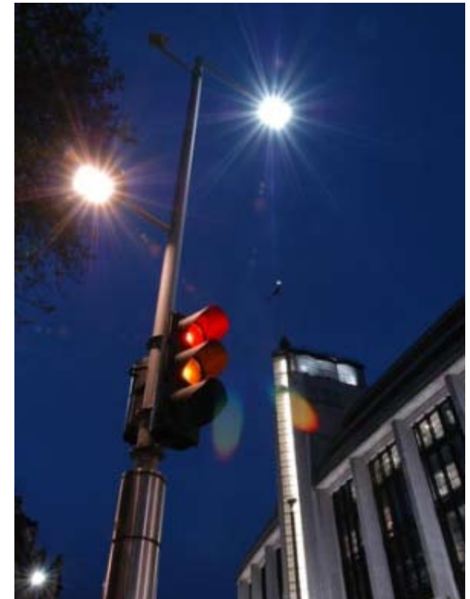
Example of combined pole usage
