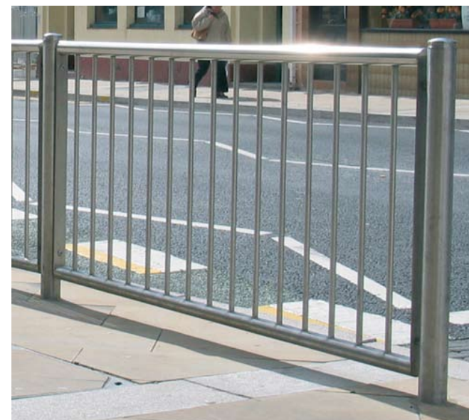
Guardrailing set 450mm back from kerb edge
