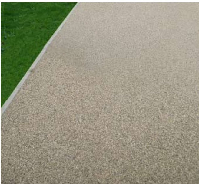
Resin bound gravel surfacing
