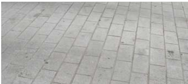
Mid-grey granite sett paving
