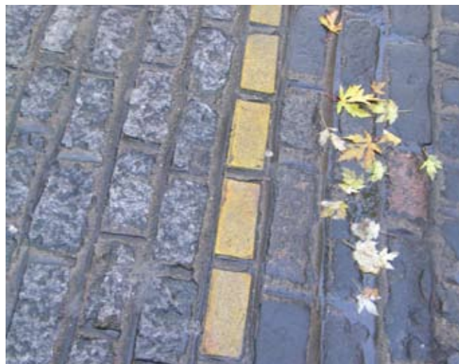
Yellow block paving for yellow lines
