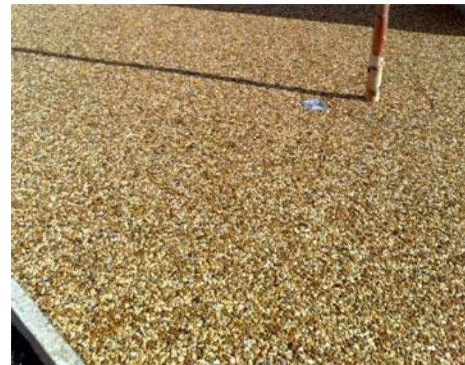
Permeable gravel paving
