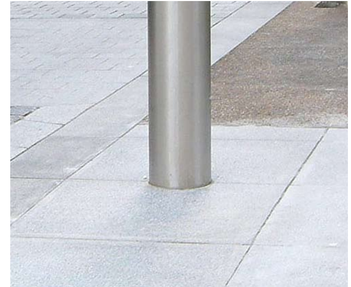
Paving slabs neatly cut to fit around bollard
