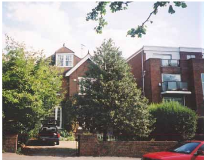
No.4 Edge Hill and the flats at No.2, outside the Conservation Area
