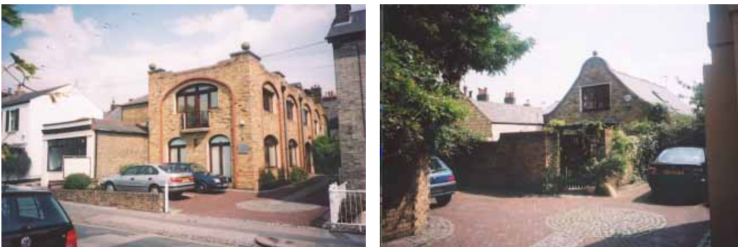
Thornton Road; Nos. 18 and 19 Thornton Road; and No. 21 Thornton Road at the rear.
