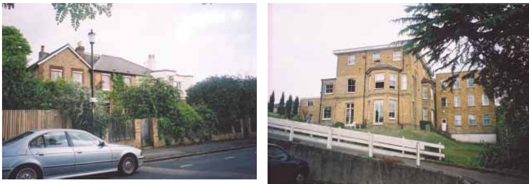
Nos. 15 and 16 Hillside, and No. 17 from the west showing the ramp to the car park
