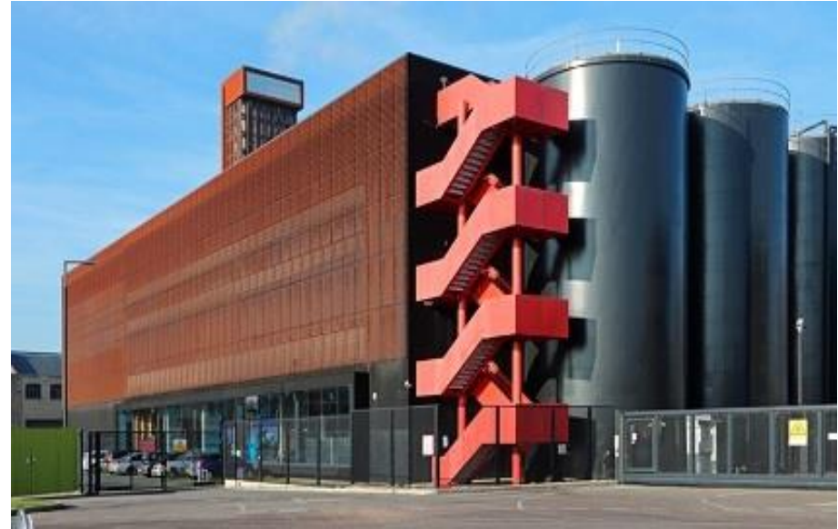
Figure 4.8 - The vast majority of large existing heat networks burn fossil fuels in an Energy Centre (through CHPs and gas boilers). In order to decarbonise, they will seek to generate a growing proportion of their heat with heat pumps. DH2 represents a network targeting a 40% proportion of heat from heat pumps.
