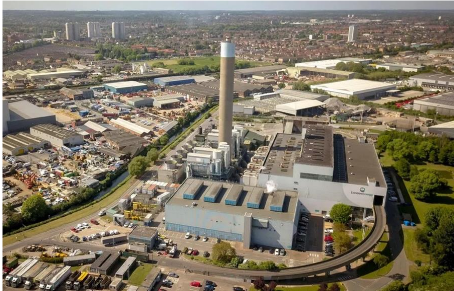
Figure 4.7 - Energy from Waste heat networks are centred around using heat that is produced by the process of waste incineration (above the North London Edmonton incinerator) distributing that heat to homes close to it or much further (Photograph: pxl.store/Alamy)
