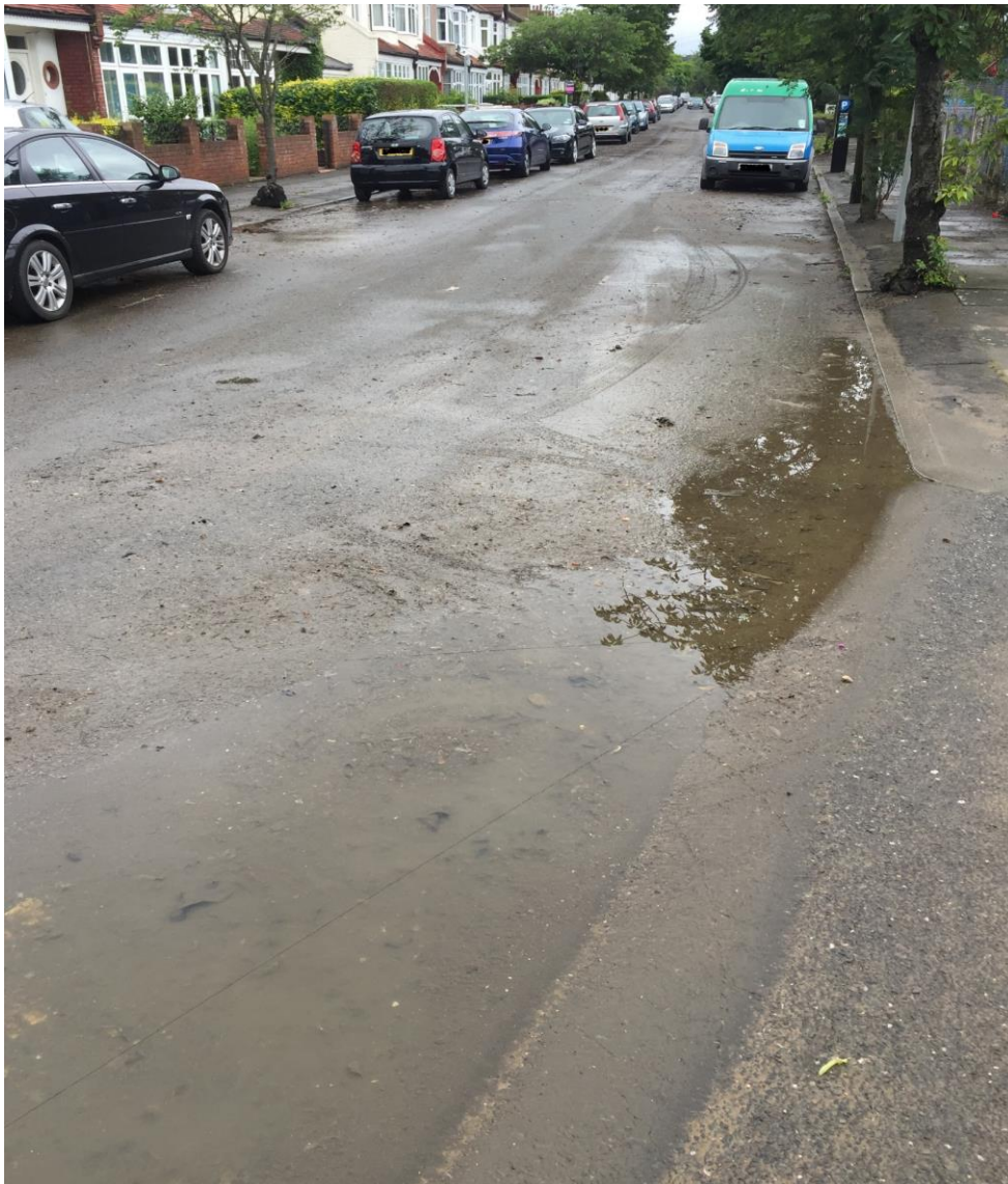
Figure 7.1: Extent of the flooding in Abbott Avenue post-June 2016 incident
