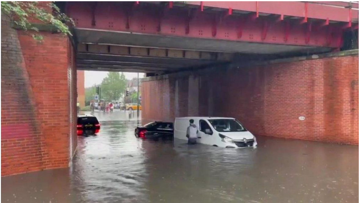
Figure 5.3: Flooding to the Approach Road underpass in Raynes Park on 12 th July 2021 (Resident’s photo submitted to Merton Council)
