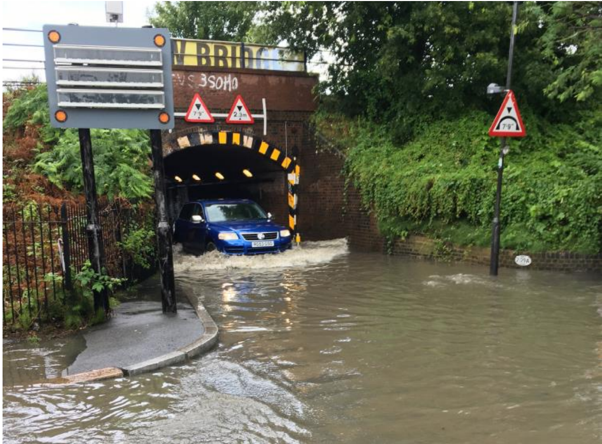
Figure 5.2: Flooding to the Lower Downs Road underpass on 12 th July 2021 (Resident's photo submitted to Merton Council)
