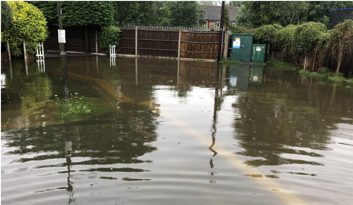
Figure 6.2: Flooding to Marina Avenue on 25 th July 2021 (Resident’s photo submitted to Merton Council)
