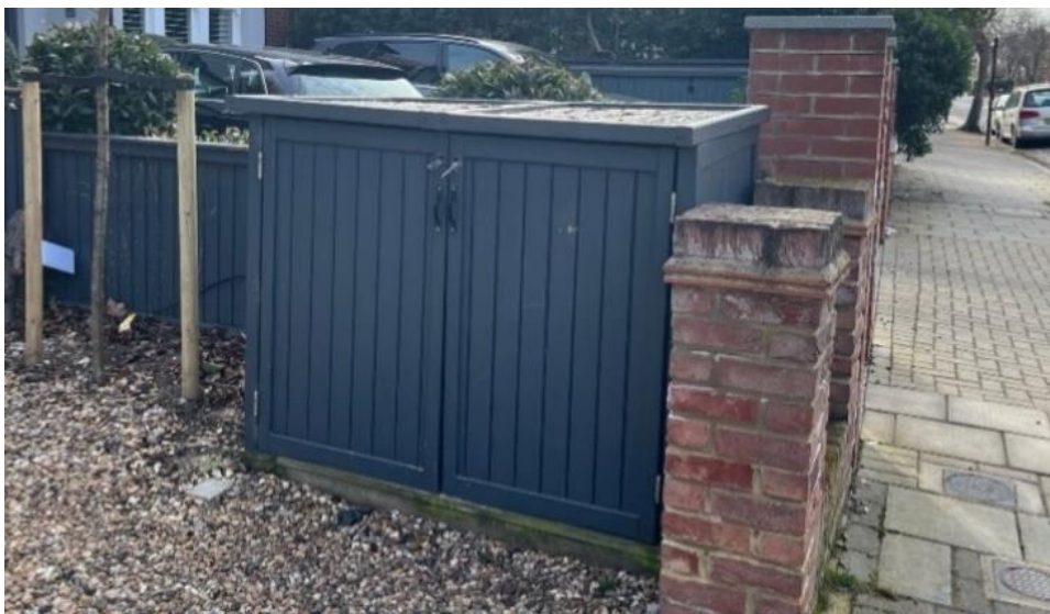
Figure 6 - External Bin Store (Front)
