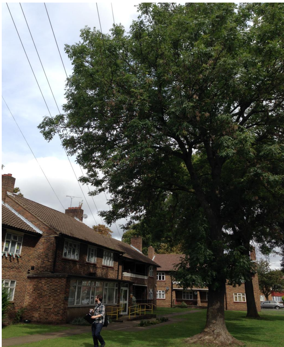
Photograph C11 – 2-18 Ravensbury Grove and Community Hall
