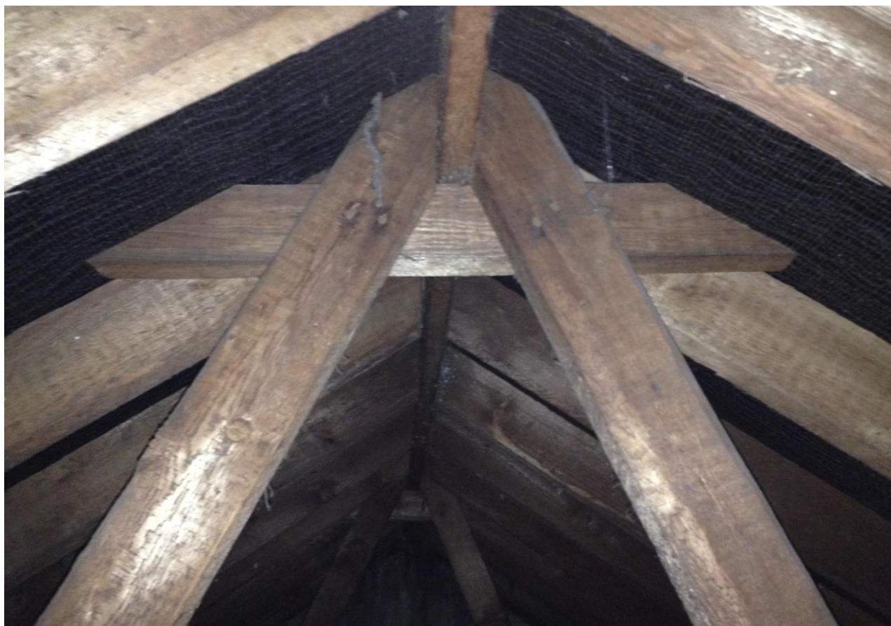
Photograph C9 – 14 Ravensbury Grove Roof Detail
