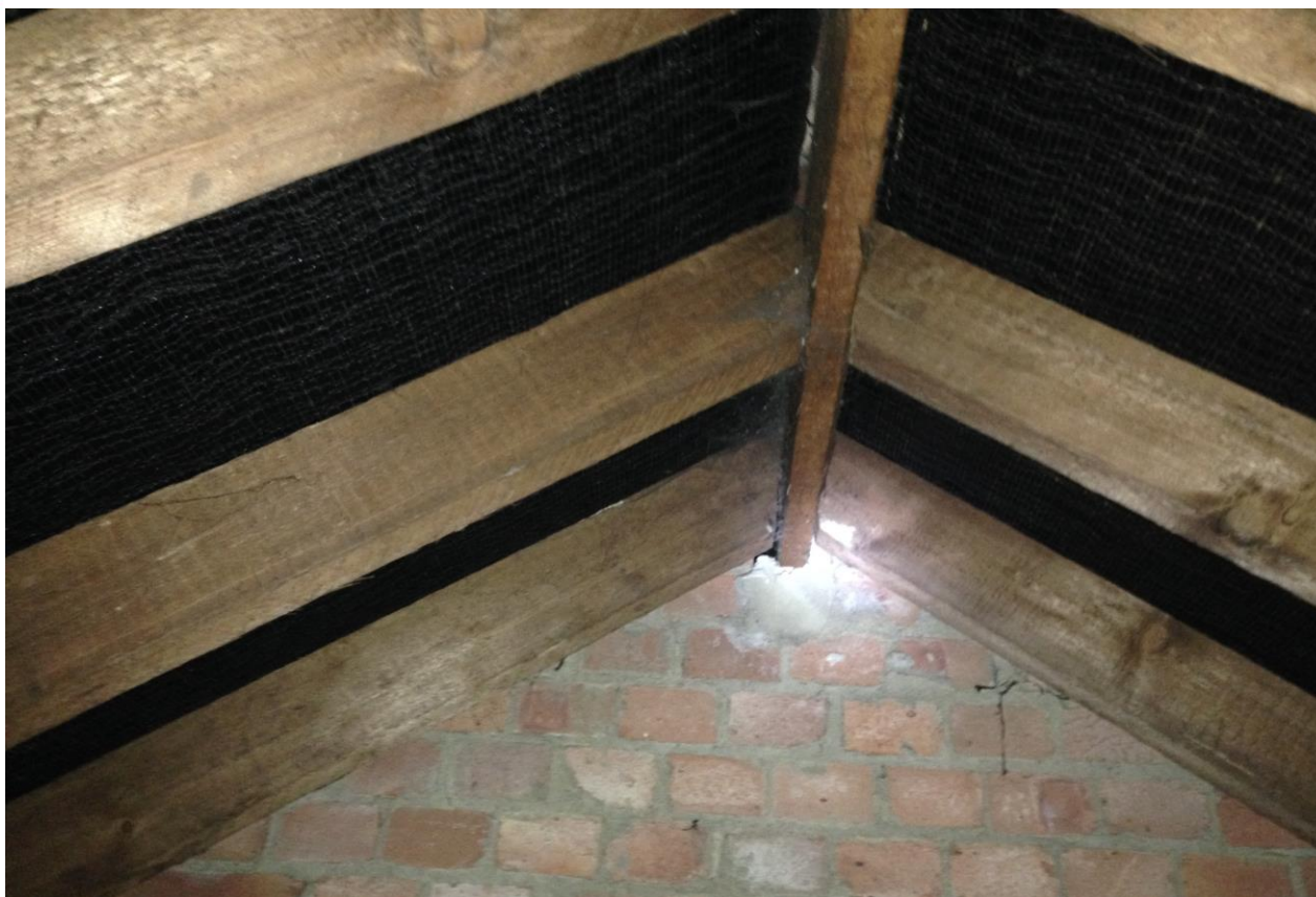
Photograph C7 - 14 Ravensbury Grove Roof Space
