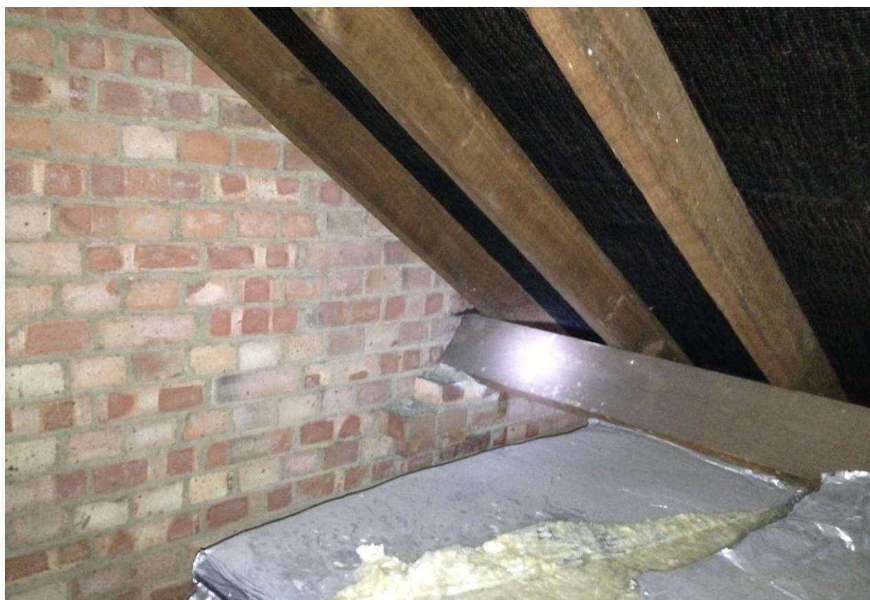
Photograph C6 – Purlin Support on Masonry Gable
