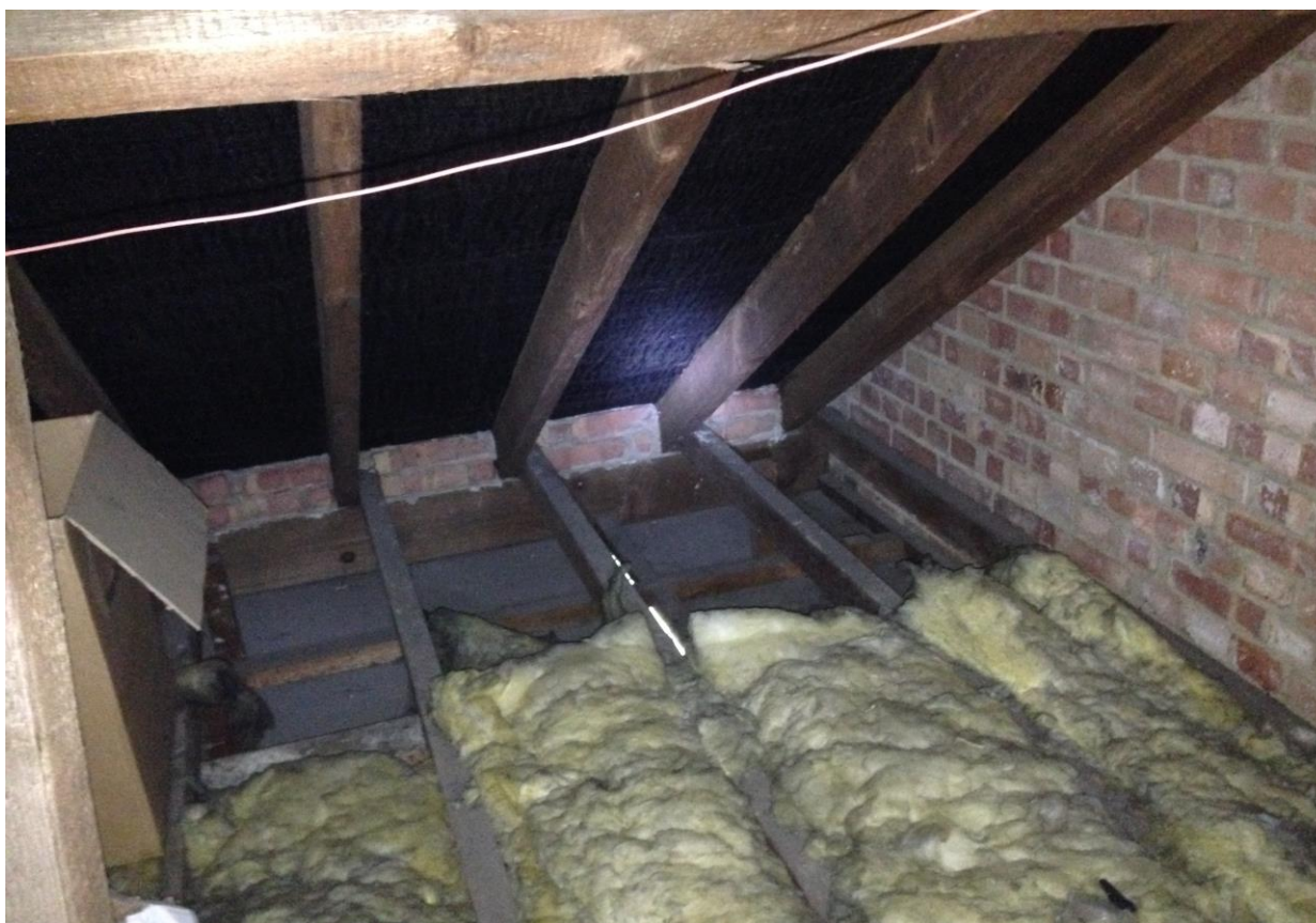
Photograph C8 – 14 Ravensbury Grove Roof Space
