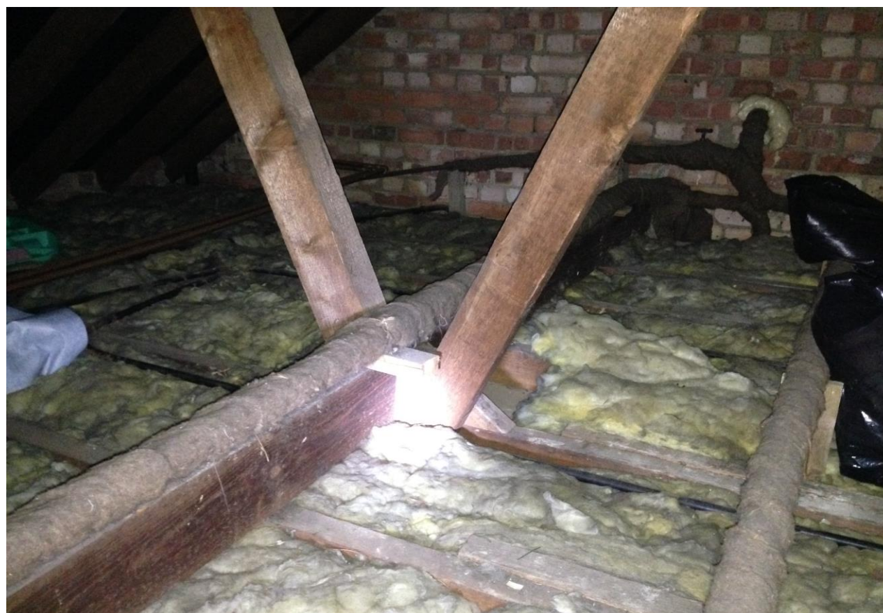
Photograph C10 – 14 Ravensbury Grove Roof Space
