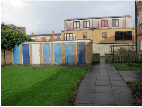
Photograph 4 – Tenants stores and communal garden to rear of block. Stores are generally in a poor state of repair
