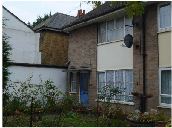
Photograph 5 – No. 60 Pincott Road – Front elevation with original Crittall type window configurations
