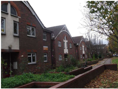
Photograph 1 – Will Miles Court
