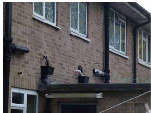
Photograph 4 – showing rear of the block and projecting single storey building
