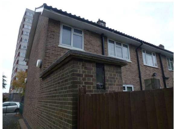
Photograph 7 – single storey rear addition.
