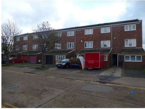
Photograph 5 – Front elevation showing projecting garages / conversion to habitable rooms
