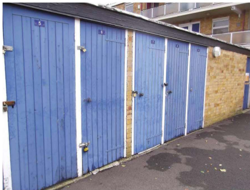
Photograph 20 – Norfolk House - external tenant stores
