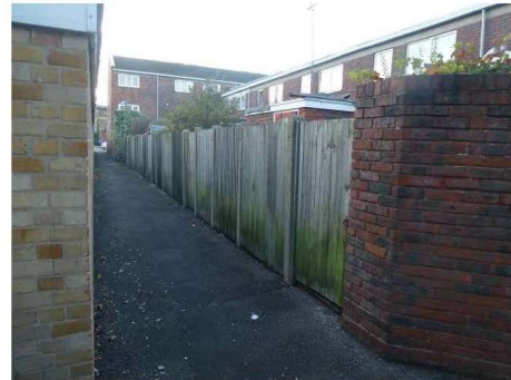
Photograph 14 – view of rear garden fences
