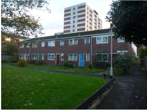
Photograph 11 - Front elevation of two storey terraced houses
