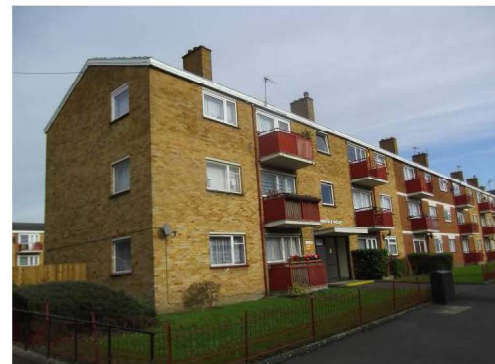
Photograph 17 – Norfolk House - Front elevation
