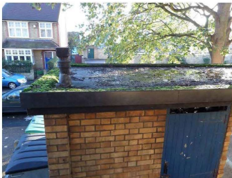
Photograph 16 – Merton Place -View of roof over refuse store
