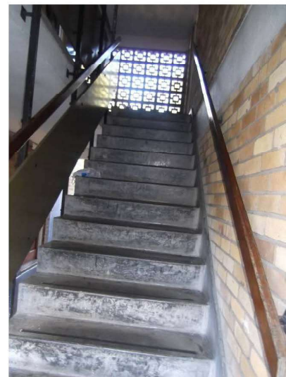
Photograph 3 – Mychell House – Typical communal staircase finishes
