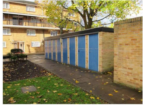
Photograph 6 - De Burgh House – External tenants stores (Merton place in the background)
