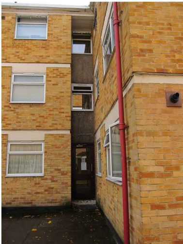
Photograph 3 – De Burgh House – Rear courtyard door
