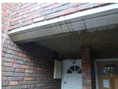
Photograph 3 – view of entrance soffit showing overhang of first floor concrete slab
