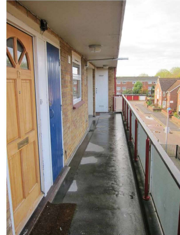
Photograph 11 – Hilborough Close Access Balcony
