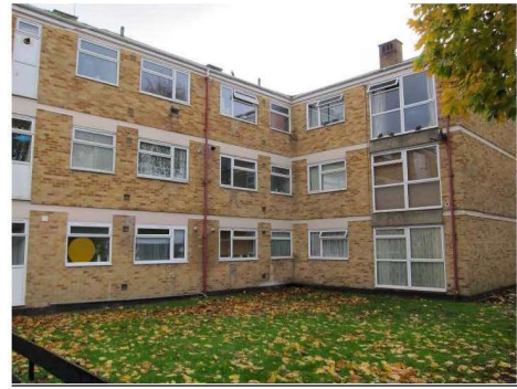
Photograph 2 – De Burgh House- Rear elevational treatment
