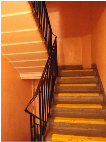
Photograph 5 – Internal communal staircase, concrete stair structure and painted metal balustrading
