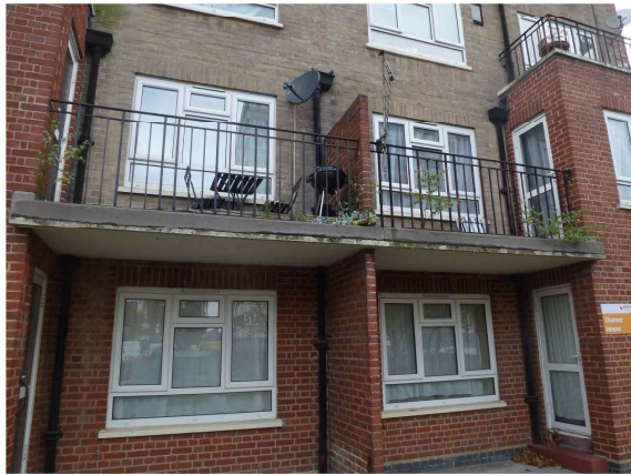
Photograph 5 – Eleanor House – private balconies
