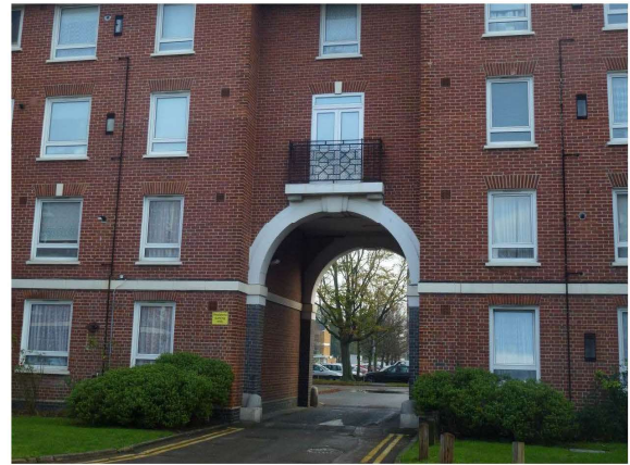
Photograph 15 - Ryder House - passageway
