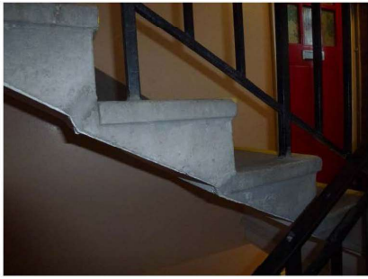
Photograph 9 – Communal staircase. Concrete stair detail
