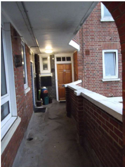
Photograph 3 - Deck access balcony to Becket Close
