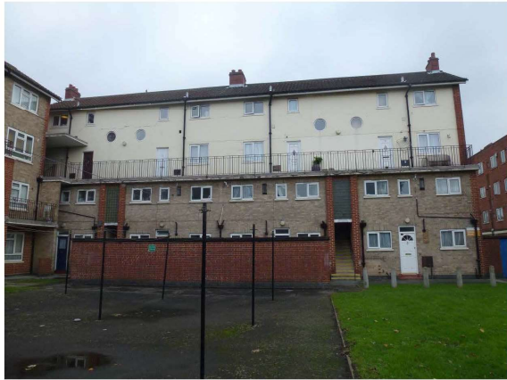
Photograph 1 – Eleanor House –Upper floor maisonettes and access balcony. Ground floor entrances to flat units
