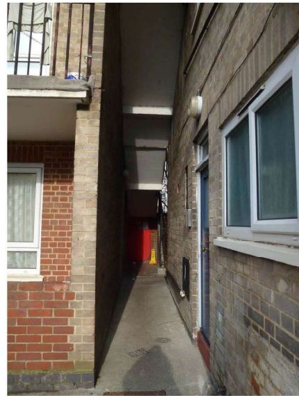
Photograph 4 – Eleanor House – passage to external communal staircase.
