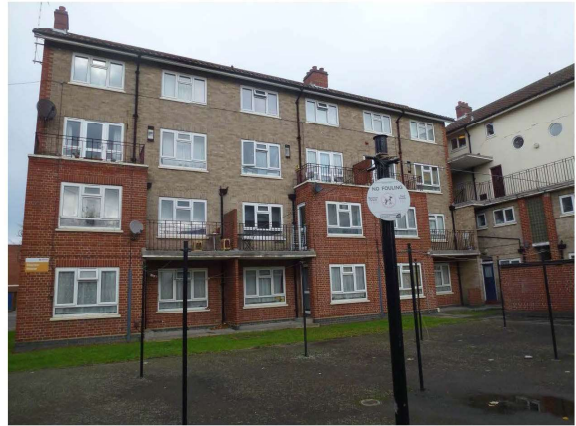
Photograph 2 – Eleanor House – Private balconies
