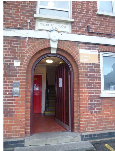
Photograph 6 – Typical entrance to communal staircase - Gilbert Close block. Doors appear to have been installed in the last 10 years. There is no level access to ground floor flats.
