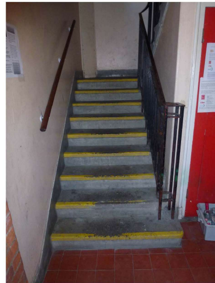
Photograph 12 – Typical view of communal stair access with services cupboard to the right of the staircase
