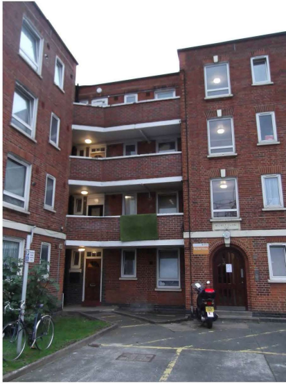
Photograph 1 – View of North communal entrance door and access balcony arrangement to Becket Close.
