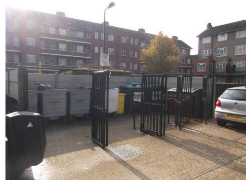
Photograph 16 – external refuse storage enclosure showing typical concrete hard standing and tarmac within the enclosure
