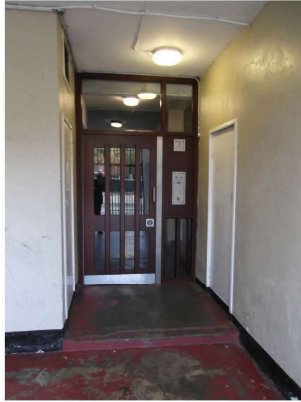
Photograph 17– secondary ground floor entrance to blocks.
