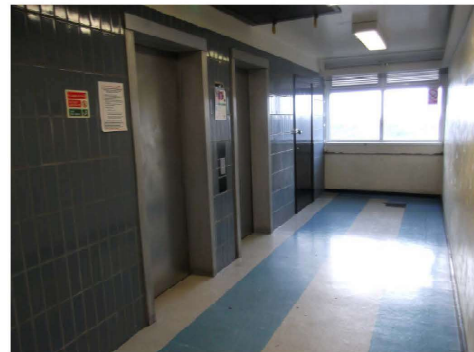
Photograph 21 – Typical lift lobby with glazed wall tiles
