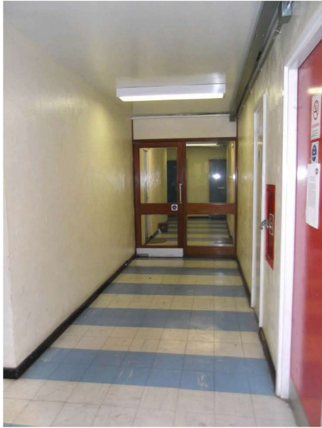
Photograph 13 – Typical upper level communal corridor for access to flats
