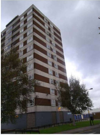
Photograph 1 – View of external view of South elevation
