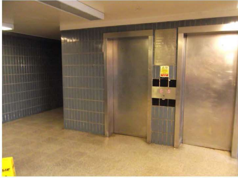
Photograph 23 – view showing typical lift lobby with stainless steel lift door surrounds and ceramic wall tile finishes.
