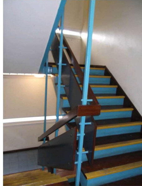
Photograph 14 – Typical view of internal communal staircase. Stairs are fitted with Hardwood treads and Handrails with hardwood lipped laminated panels to form balustrade
