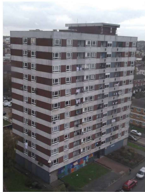
Photograph 18 – Hudson Court as viewed from roof of May Court
