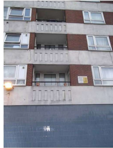
Photograph 2 – Typical private balconies
