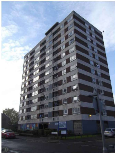
Photograph 5 – May Court as viewed from the North East.
