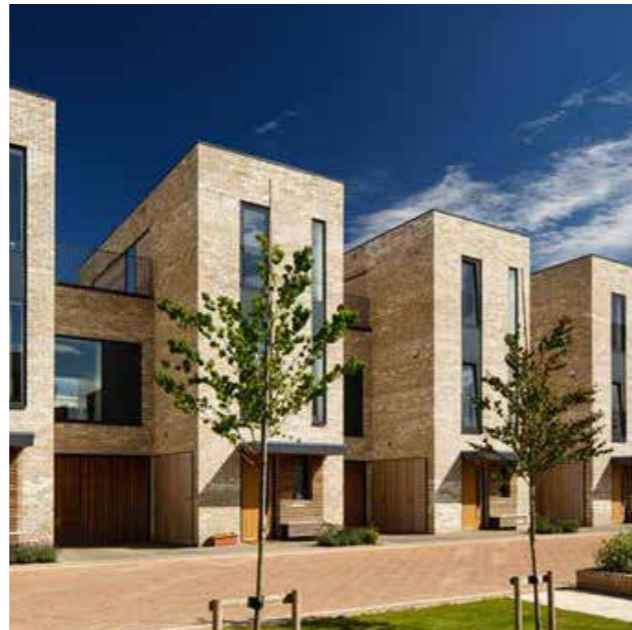
Precedent: Mews individually expressed with articulations in the facade and entrances
