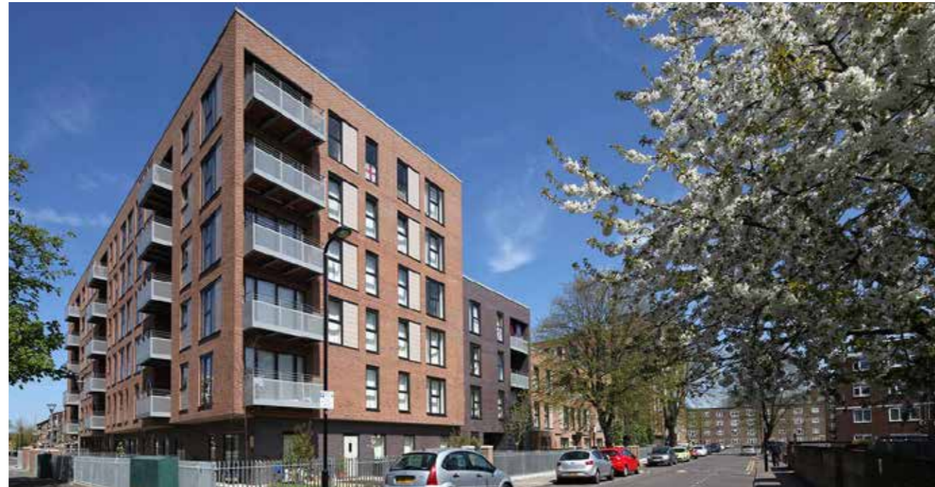
Precedent: variation in roof heights and strong corners at entrances
